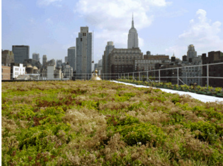
Figure 2.1. Extensive Green Roof on the Cook + Fox offices, New York, New York.
