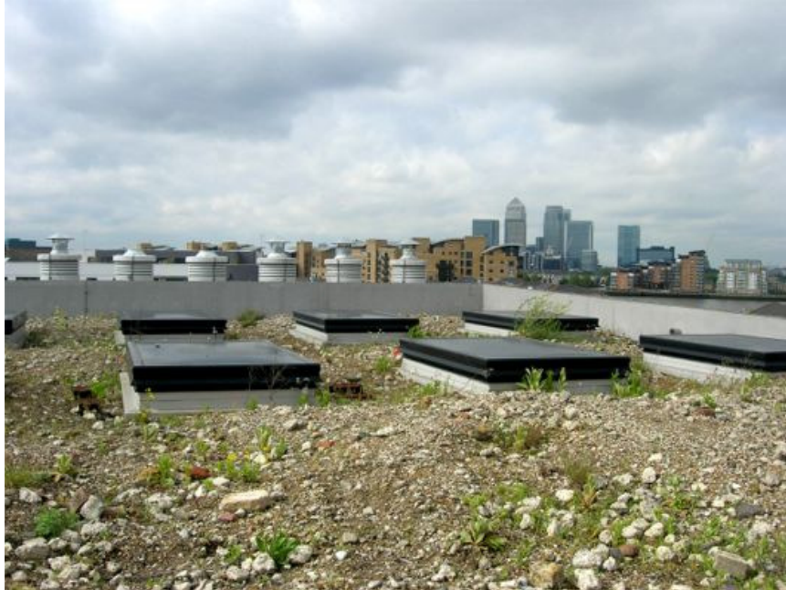
Figure 2.4. Brown Roof on the Laban Dance Center, London, England, UK.
