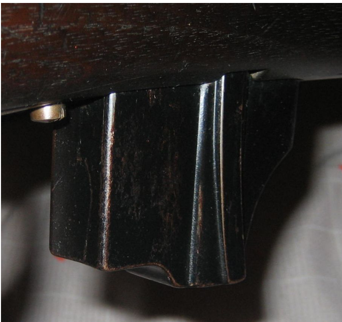
Figure 11: Four-Round Vitali Box Magazine
