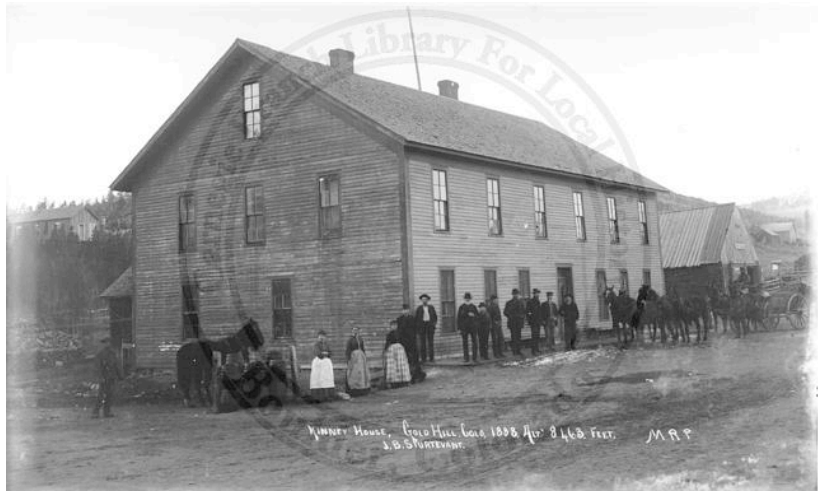
Fig. 3: The Grand Mountain Hotel, constructed by Charles Wentworth. This photo was taken July 4, 1886 by J.B. Sturtevant. (Courtesy of the Carnegie Library for Local History—Boulder, Colorado).
