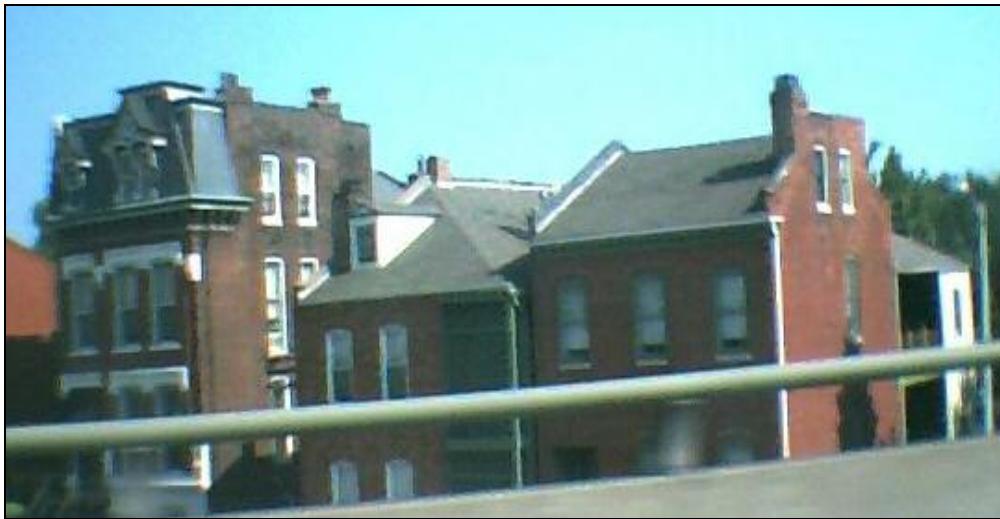
Fig. 28: Evidence of St. Louis's Decay. Though these buildings may have been serviceable when built in the nineteenth century, they now serve as a symbol of St. Louis's decline, especially as many buildings similar to those illustrated above are boarded up and are fire hazards.
