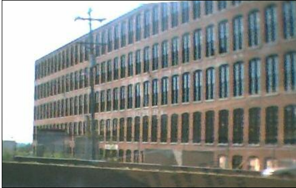
Fig. 21: An abandoned warehouse by the waterfront; a remnant, not yet demolished (as of 2005), of St. Louis's industrial past. Buildings such as this demonstrate why the elites moved far away from the industrial core.
