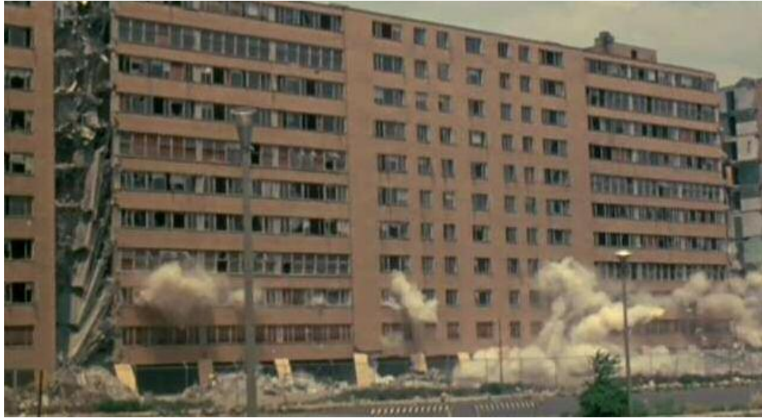
Fig. 34. Dynamite Explodes a Building in Pruitt-Igoe. Source: http://www.spiritofbaraka.com/
