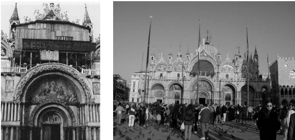
Illustration 5: St Mark's Cathedral, Venice. Photos of the west façade after restoration. Photographs courtesy of www.historylink102.com .
