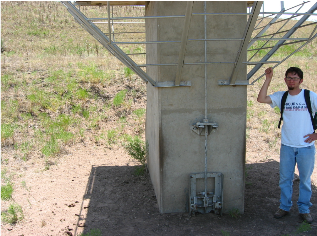
Figure 3. Chris Ennen investigates sediment at riser as a result of livestock trampling
