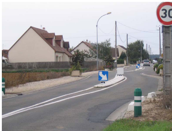
Figure 2. Chicanes in Saint-Sulpice, France are used to reduce speed (Larsen 2007).
