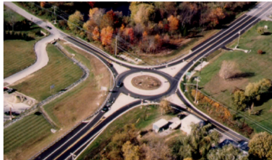
Figure 1. An example of a roundabout in Cecil County, MD (Persaud et al. 2000).
