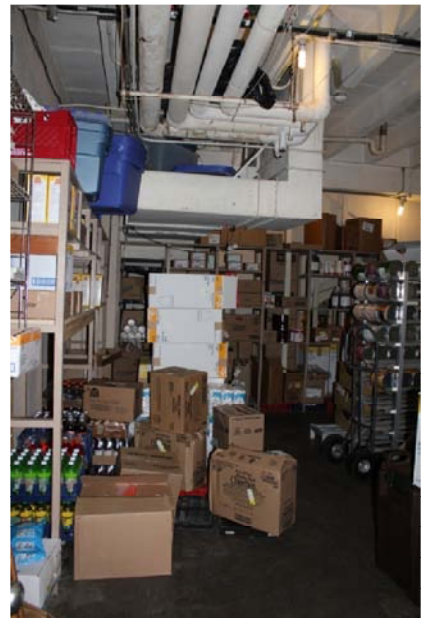
Dry Storage Room, Ceiling open to structure
