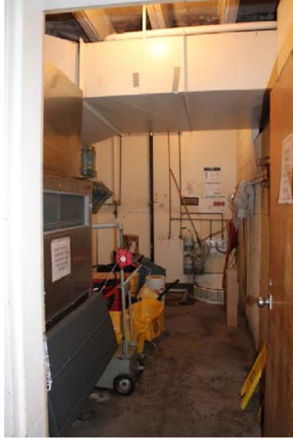
Mop Room, Ice Machine to left of image
