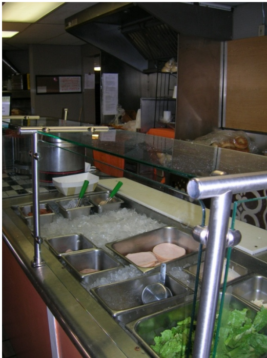
Deli Cold Service Counter, Unused Vent Hoods in Back of Photo
