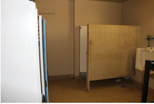
Mens Restroom Toilet, Lockers to left
