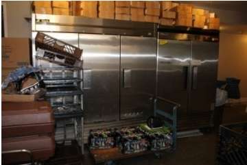
Back Dock, 3 Reach In Coolers, 2 Reach In Freezers, Energy Star Rated-Maintain in Facility
