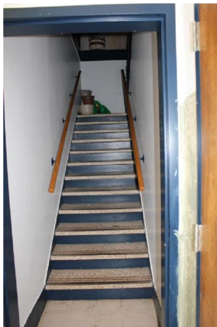
Staircase behind emergency access door
