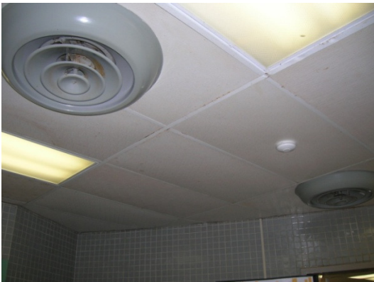
Bakery Prep area ceiling
