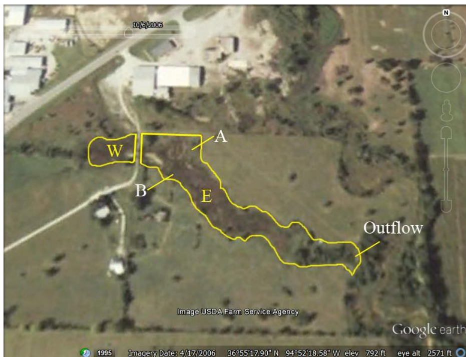
Figure 1 Aerial photo of Commerce wetland taken in 2006 (Google Earth 2013). W = West Marsh, E = East Marsh, A and B indicate seeps, Outflow was the final sampling point.
