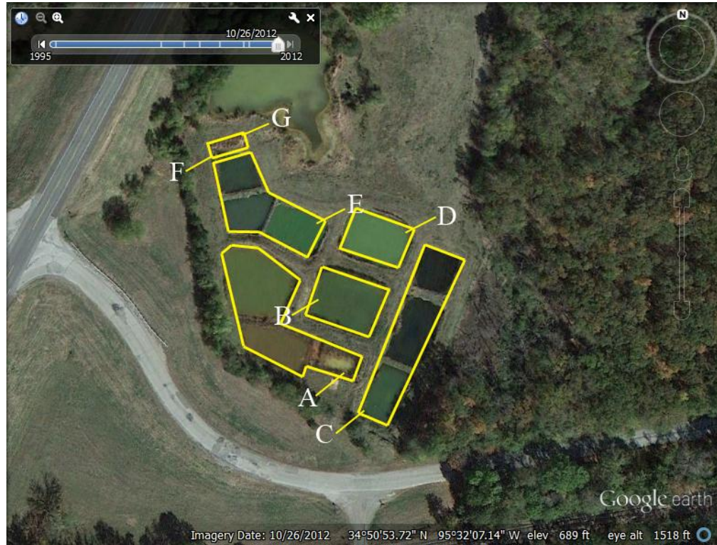
Figure 5 Aerial photo of the Hartshorne passive treatment system (Google Earth 2013). Each letter represents a sample point for each outflow as follows A=VALD, B = Ox1, C = VFW1, D = Ox2, E = VFW2, F = Ox3, G = PolWL.
