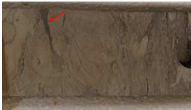
C7-001: Mud injection, sharp change from clean to mottled texture
