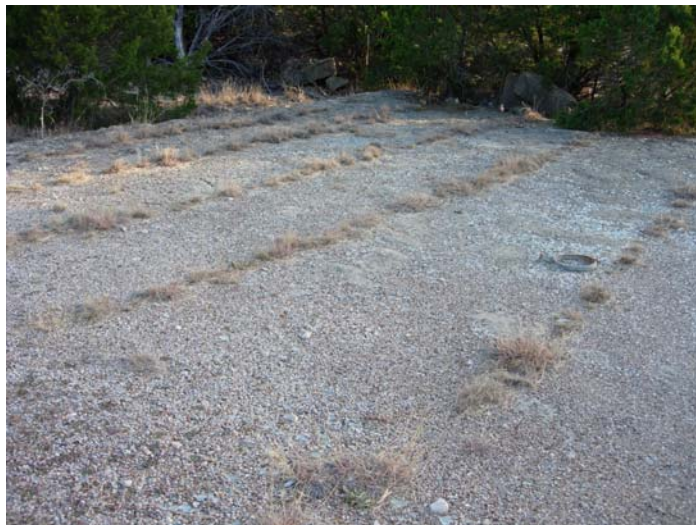
Figure 22: Fractures at PK4, with vegetation growing in fracture planes.
