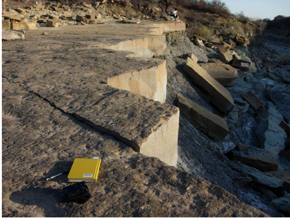
Figure 27: An image of Unit 13 and the fracture sets that form the ledge at the Brownwood Spillway
