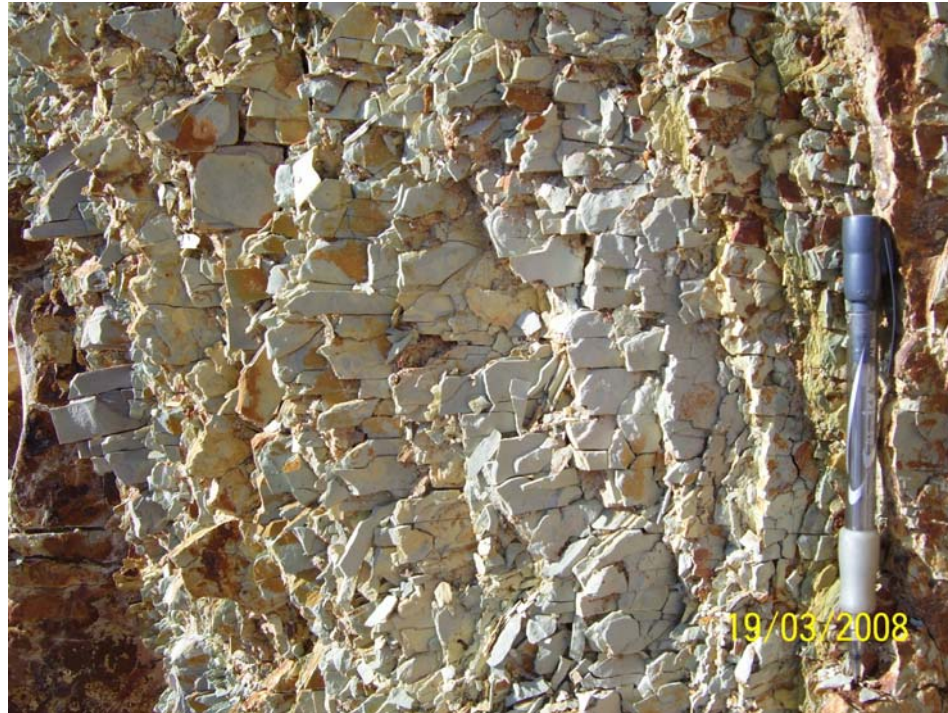
Figure 90. Densely fractured clayey units within the Arkansas Novaculate.
