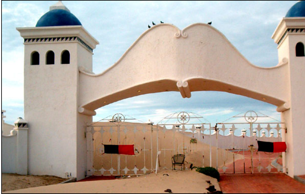
Figure 1. Sand encroachment over a retaining wall of a beach resort. C.T. Adcock image, Las Conchas, Mexico 2004.
