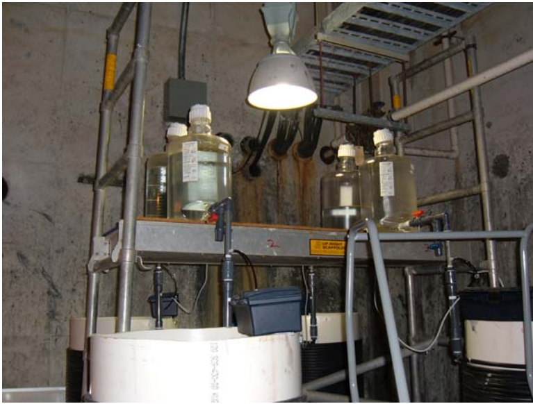
Figure 5: Scaffolding with carboys on top
