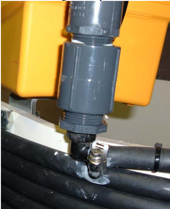
Figure 11: Static mixer connection to irrigation tubing
