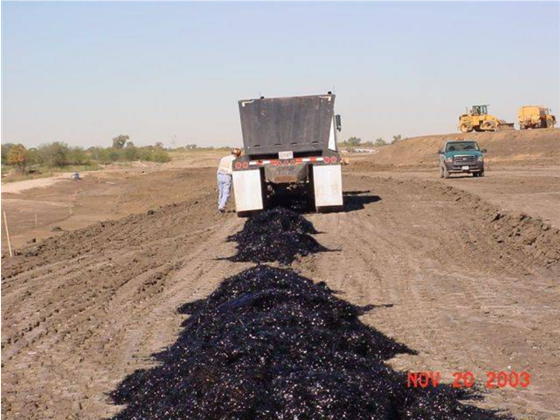
Figure 50. Spreading Fibers for FRS on PGBT Project
