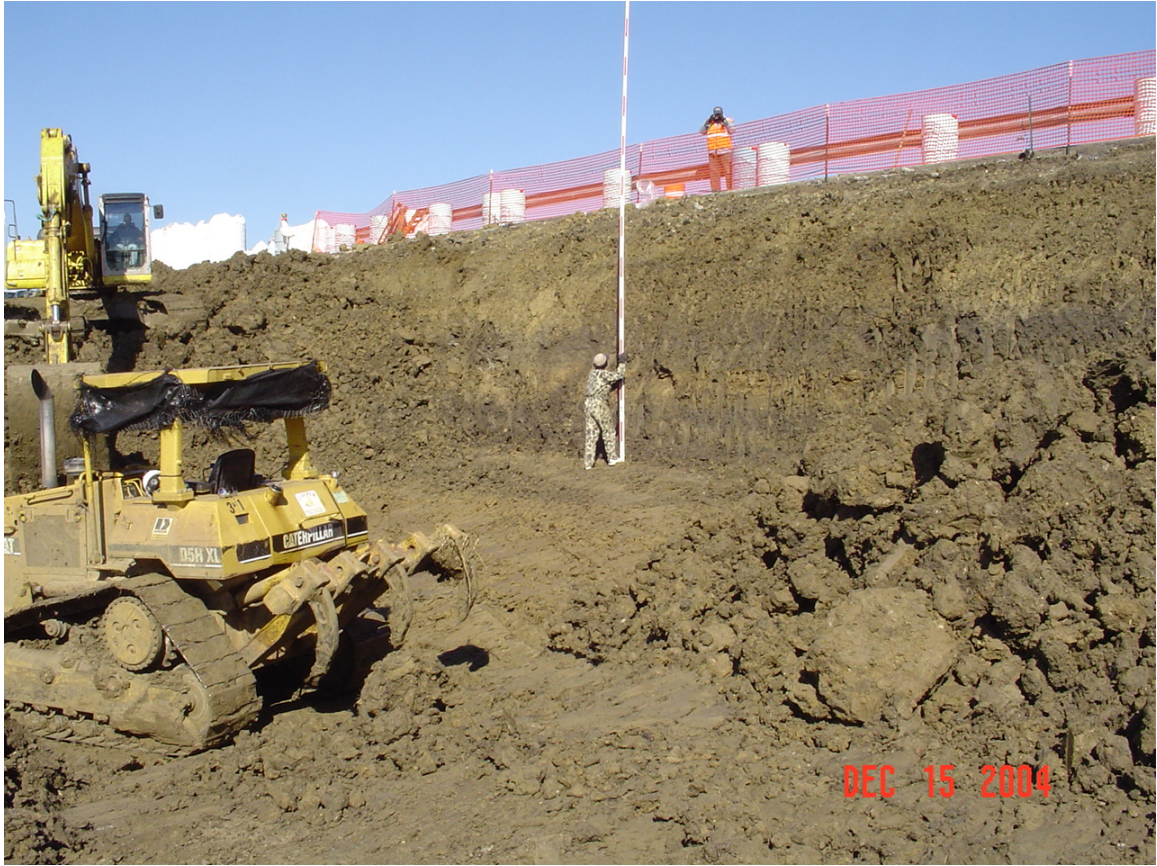
Figure 58. Initial Excavation for FRS Slope Repair – Lake Ridge Pkwy
