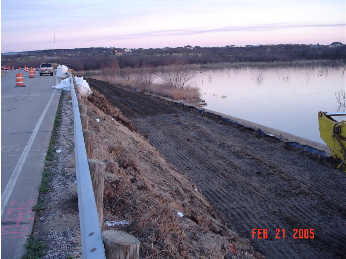
Figure 60. FRS Embankment Construction- Lake Ridge Pkwy
