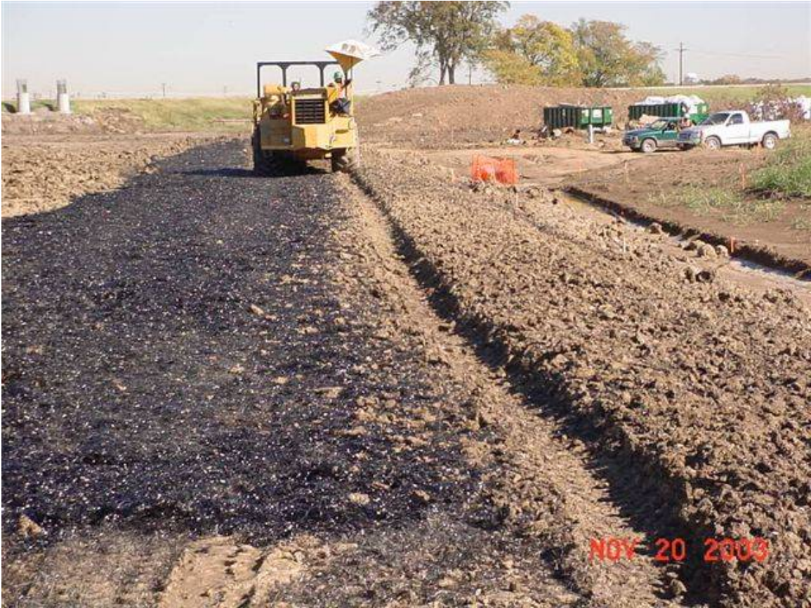
Figure 51. Mixing FRS on PGBT Project
