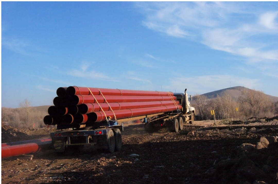
Figure 51 – Pipe Being Transported Along the Project’s Right-of-way
