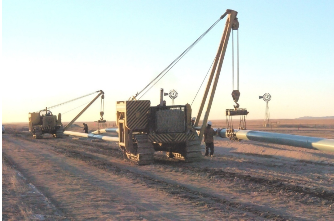
Figure 62 – Lowering-In the Pipeline
