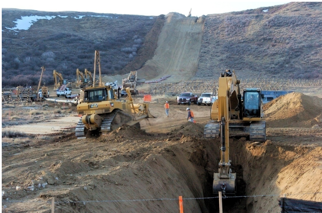
Figure 59 – Trenching with a Backhoe
