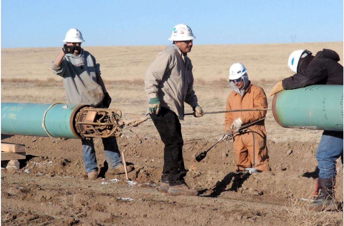
Figure 54 – Pipe Being Lined up for Welding
