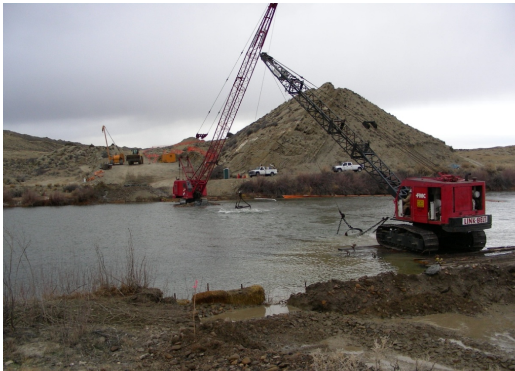
Figure 61 – Trenching a Stream Crossing with Cranes and Drag Lines
