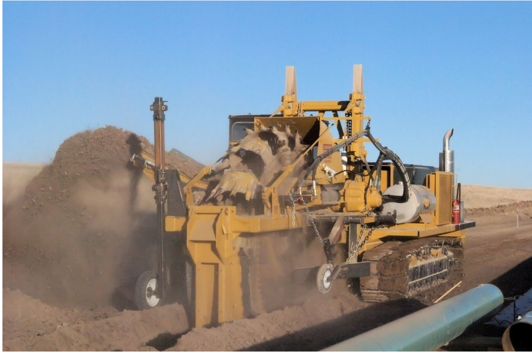
Figure 58 – Trenching with a Wheel Trencher
