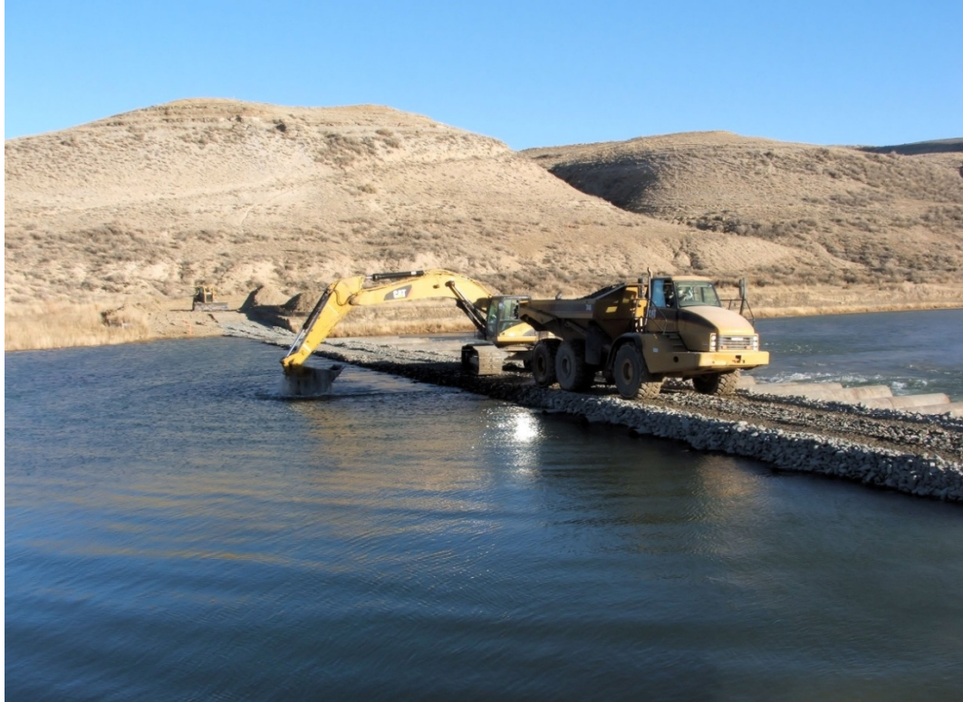
Figure 60 – Trenching a Stream Crossing with a Backhoe
