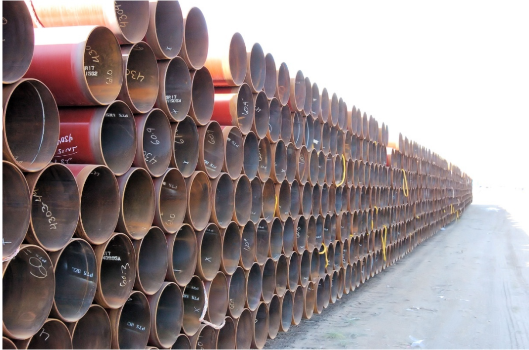
Figure 50 – Pipe Stacked Prior to Stringing
