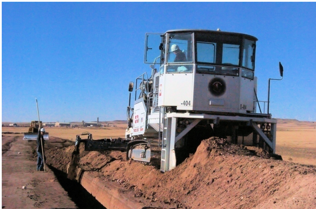
Figure 65 – Pipeline Being Backfilled
