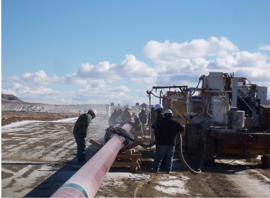
Figure 56 – Coating Field Welds with Fusion Bonded Epoxy Coating
