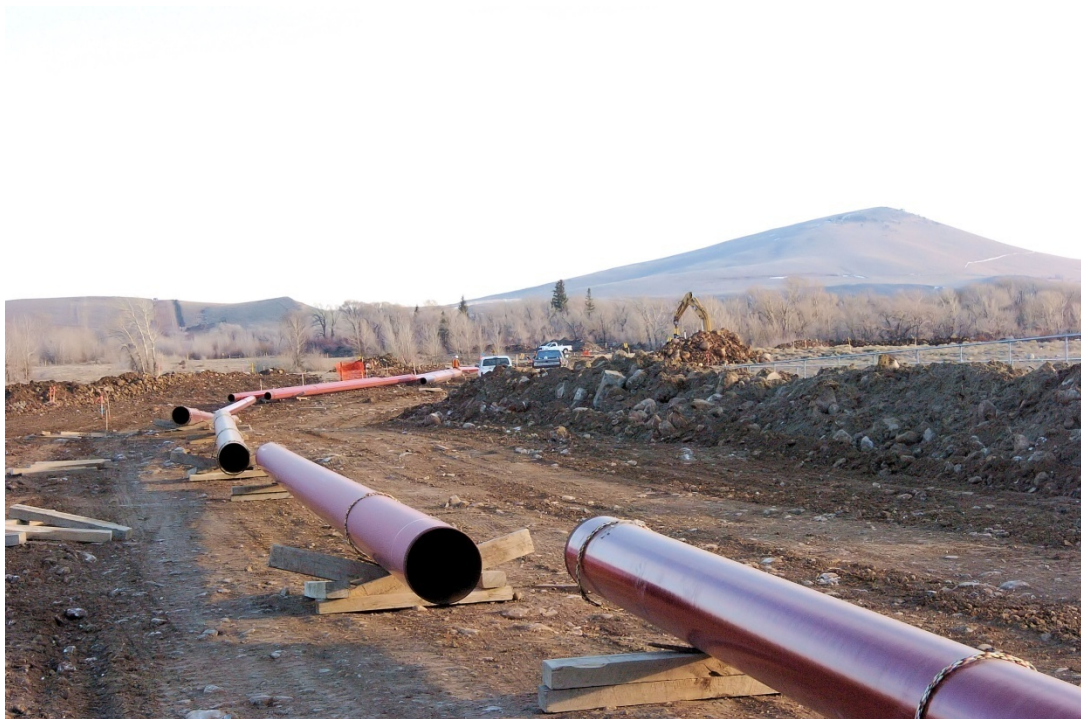
Figure 53 – Pipe Strung Along the Length of the Project
