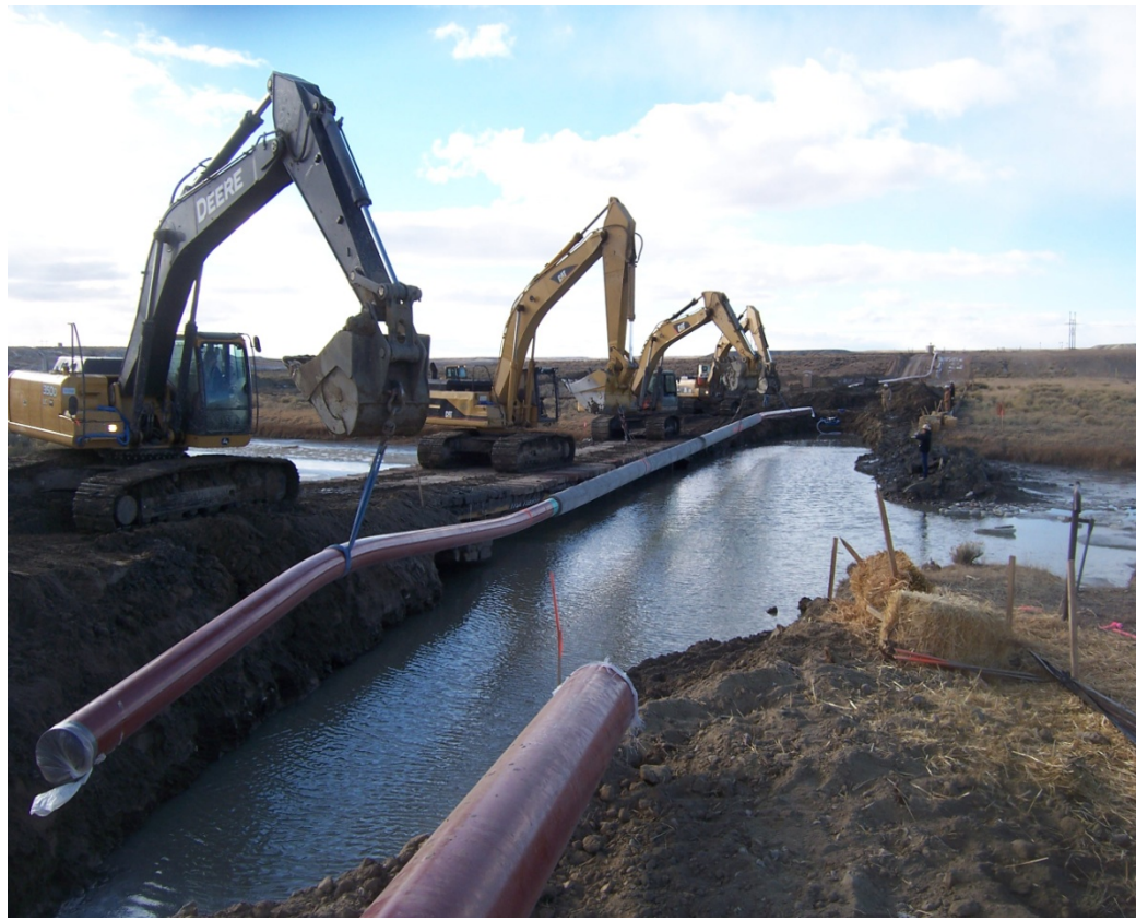
Figure 63 – Lowering-In a Stream Crossing with Portions of Concrete Coated Pipe
