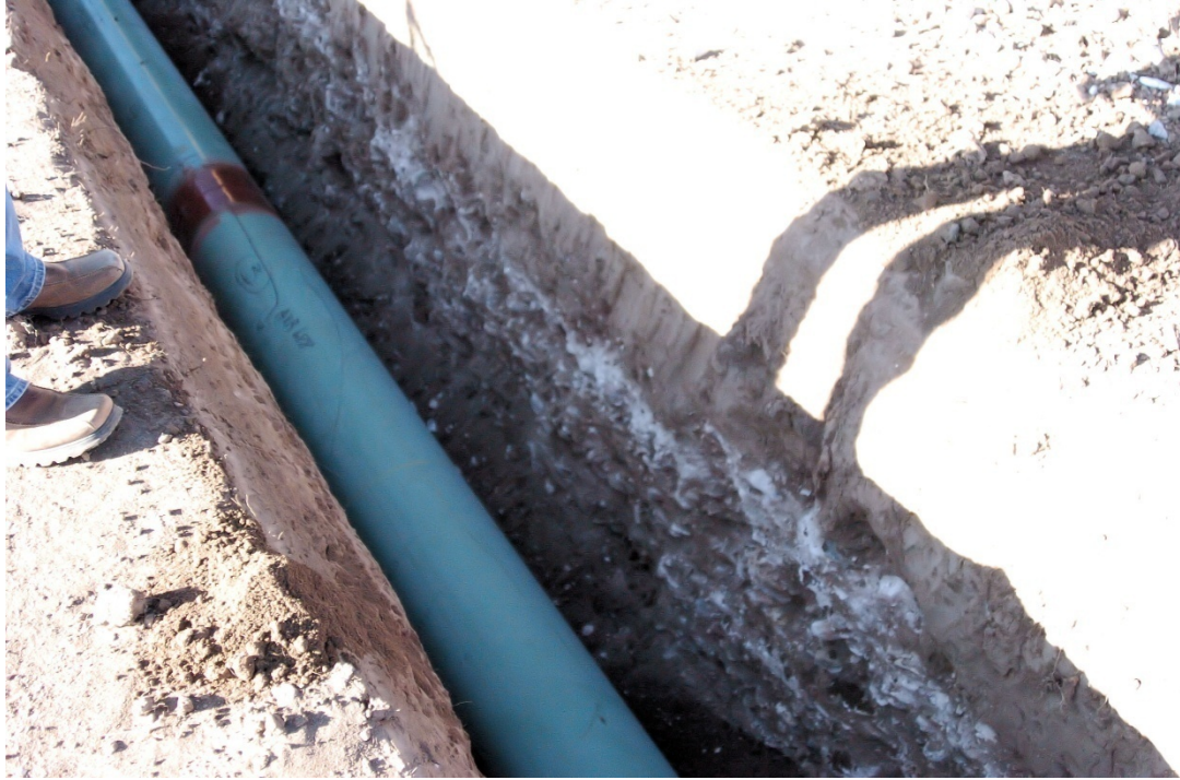
Figure 64 – Pipe Lowered into the Ditch
