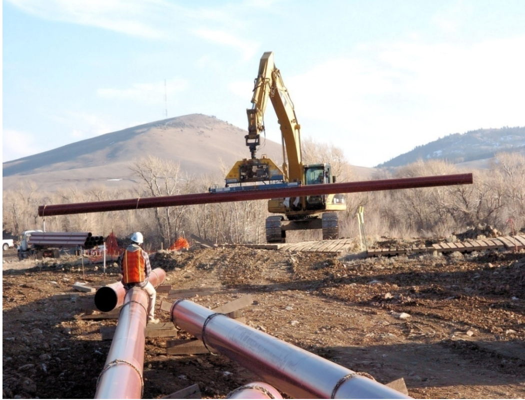
Figure 52 – Stringing Pipe Along the Length of the Project
