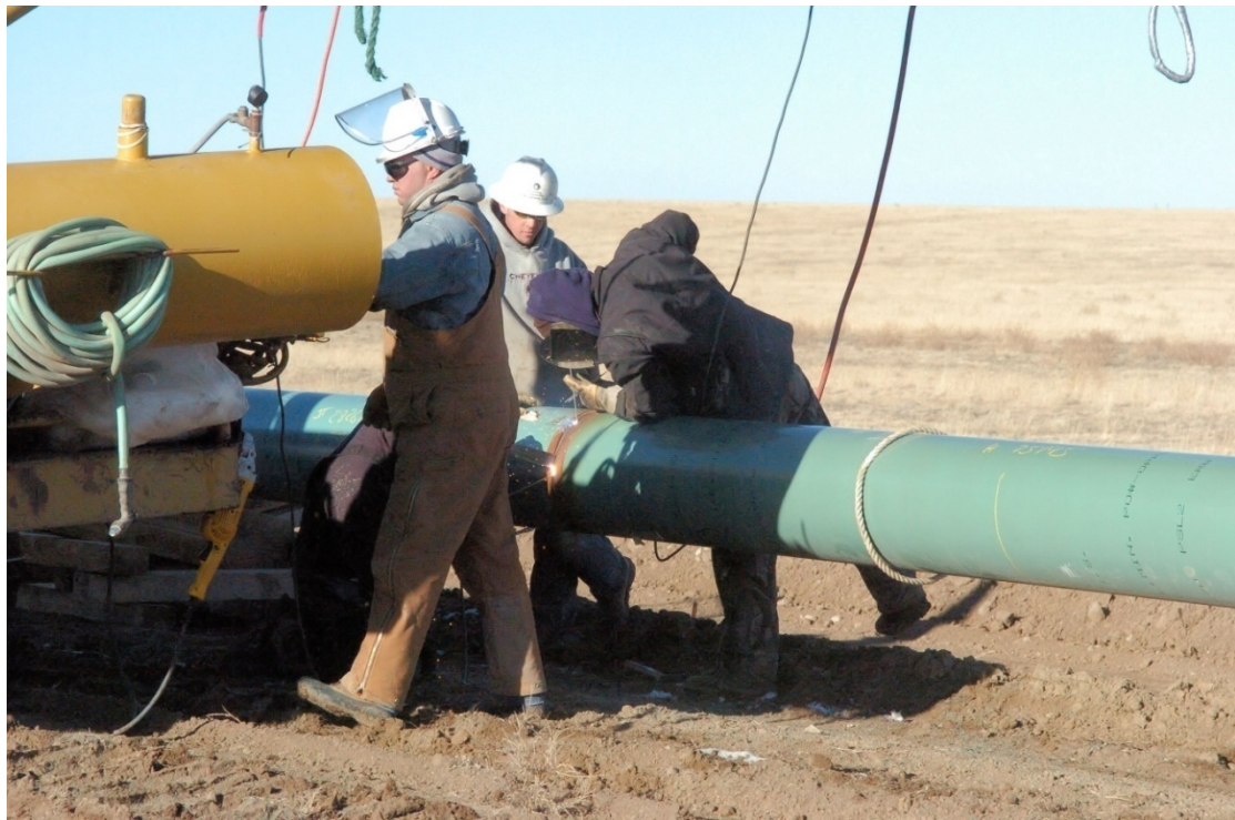
Figure 55 – Welding Crew Welding a Pipe Joint
