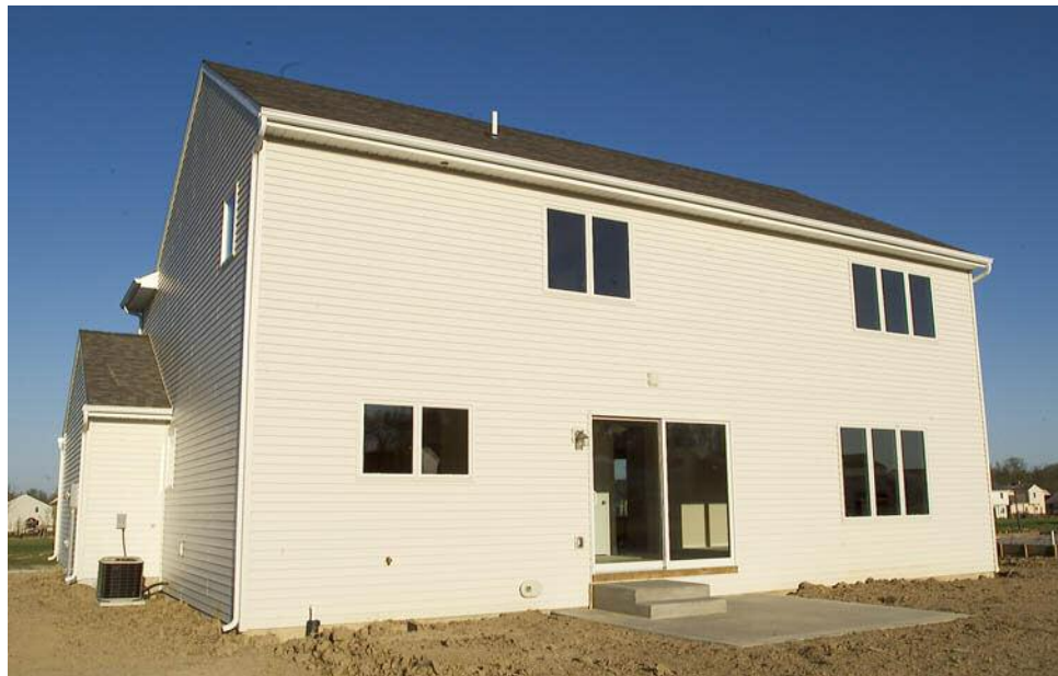
Figure 6-1(b). Back view of the house in Ft. Wayne, Indiana (Wilcox 2004)
