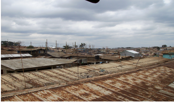
Figure 9. Rooftop view of the crowded slum.
