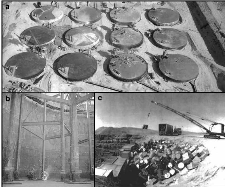
Figure 1.1 Photos depicting different waste storage methods; a) and b) show underground liquid waste tank construction while c) shows shallow burial of sealed drums (from www.hanford.gov ).
