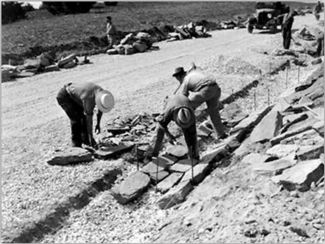
Figure 28 – Public Works project on the Blue Ridge Parkway, Virginia, 1938. (Photo 000265, NPS-HPC)
