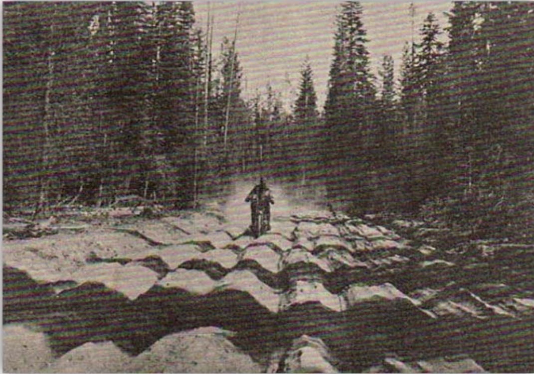
Figure 18 – Crater Lake West Entrance Road, 1910s. The volcanic soils produced voluminous amounts of dust in the summer and were nearly impassible during wetter seasons. From SOHS.
