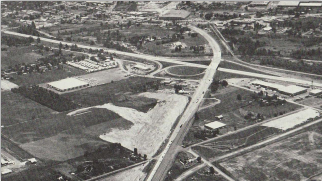
Figure 53 – Crater Lake Interchange with Interstate 5, 1966. Interstate 5 crosses the photograph from left to right; the Crater Lake Highway crosses I-5 and curves towards downtown Medford at the top of the picture. The image is oriented to the southwest (from Atwood and O’Harra, Medford 1885-1985 , 105).
