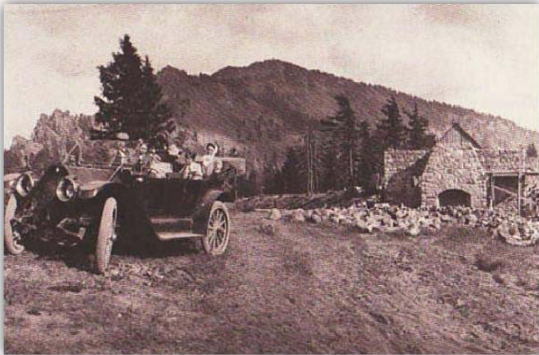
Figure 17 – Crater Lake Lodge under construction, 1910s. CLNP Archives.
