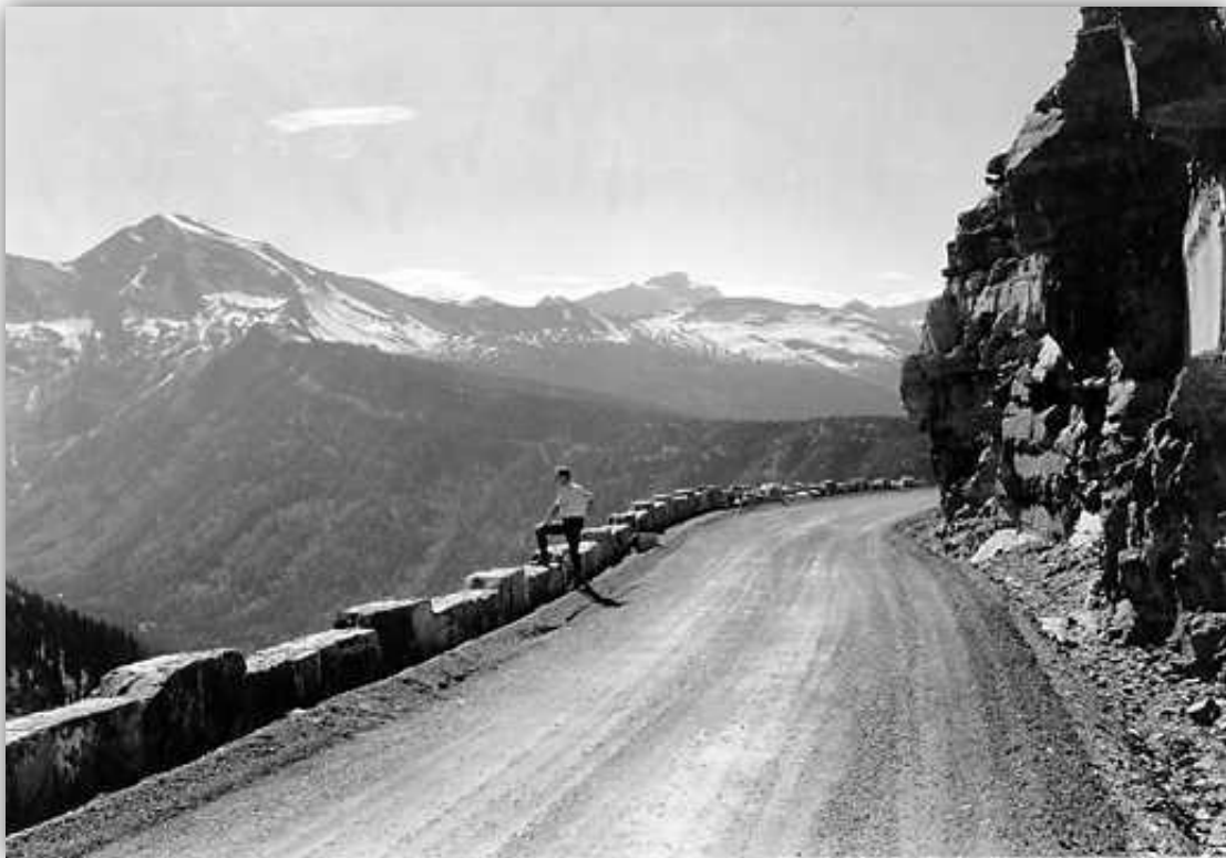
Figure 25 – The Going-to-the-Sun Road, Glacier National Park, 1932. (Photo 000034, NPS-HPC)
