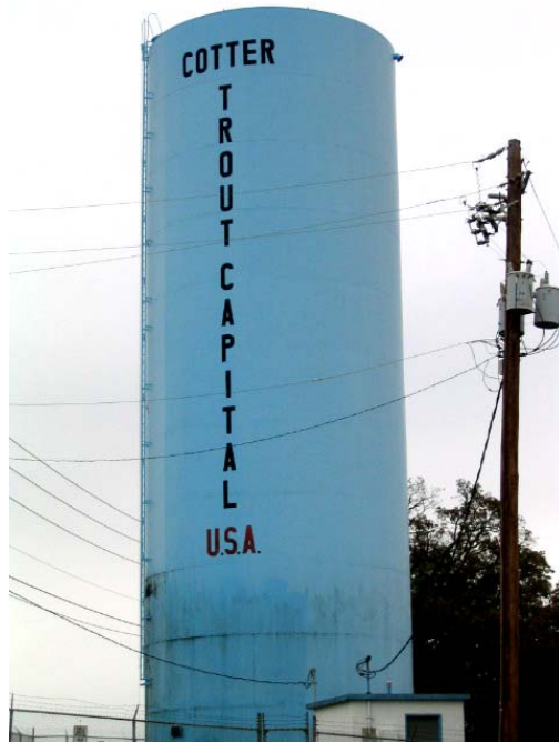
Figure 24. Cotter, Arkansas' water tower.
