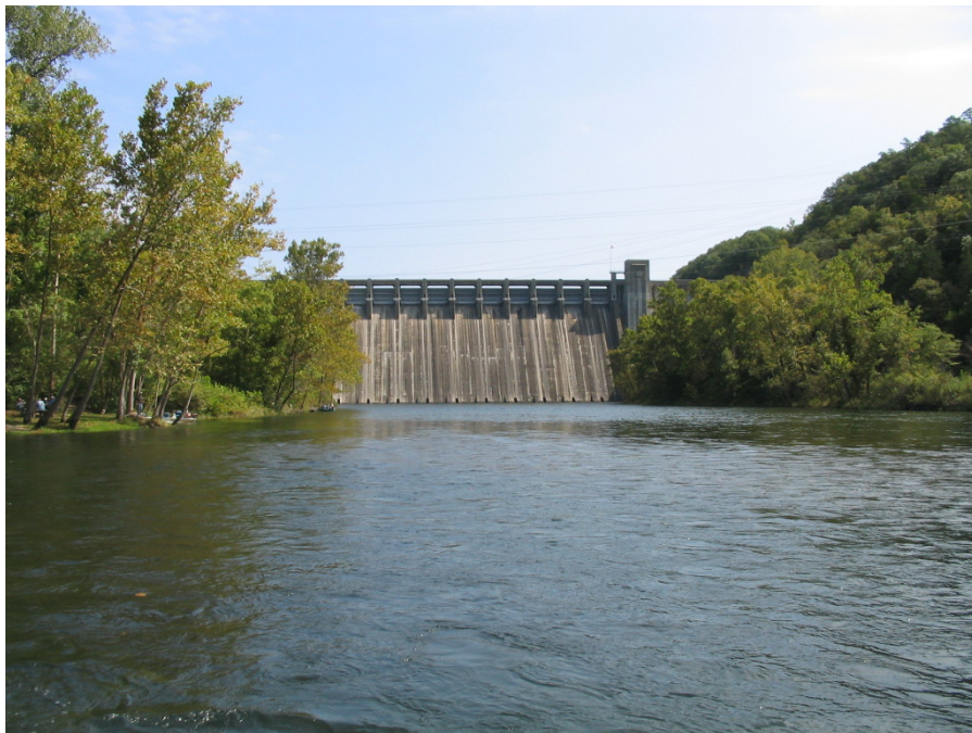
Figure 4. Norfolk Dam and tailwater.
