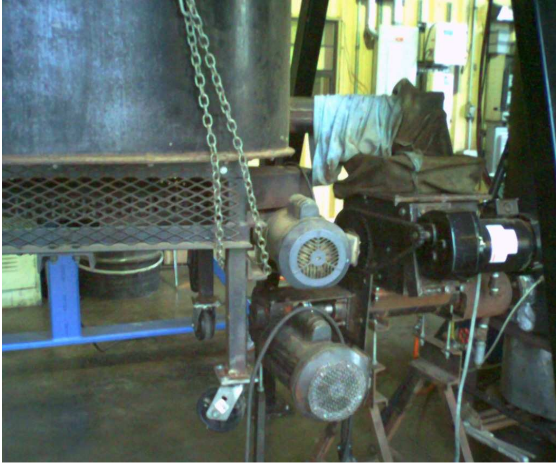
Figure 2.4 Upgraded feeding system
