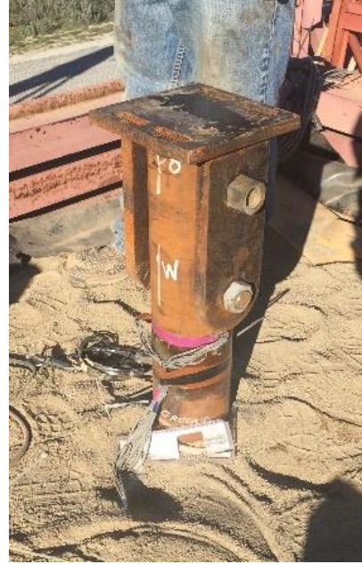
Figure 19: Installation of Grouped Pile Caps
