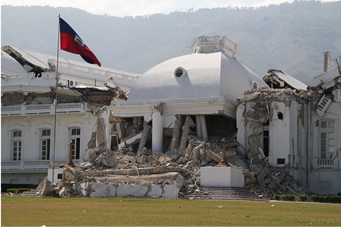
Figure 2.1 Collapsed Haiti Presidential Palace (Filter The Feed 2016)
