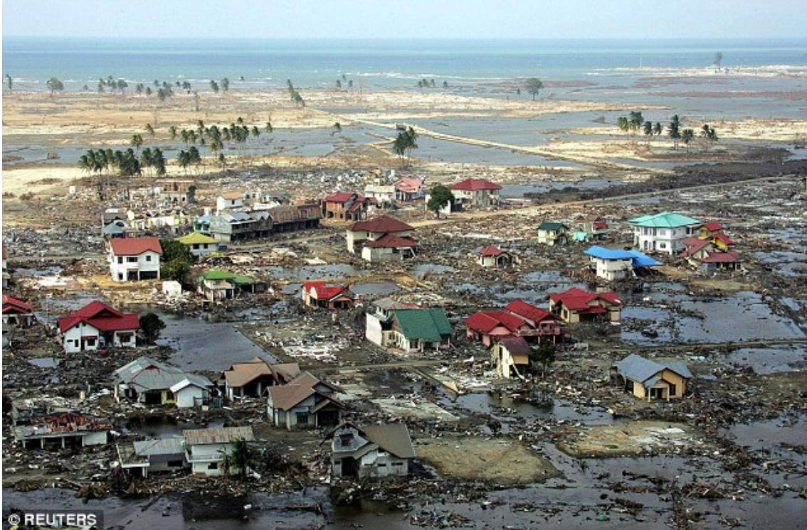
Figure 3.5 Damage in Aceh Province, Sumatra - 2004 Earthquake and Tsunami (Reuters 2005)
