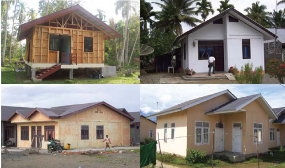
Figure 5.4 DEC housing reconstruction Banda Aceh Sumatra (de Silva 2010)
