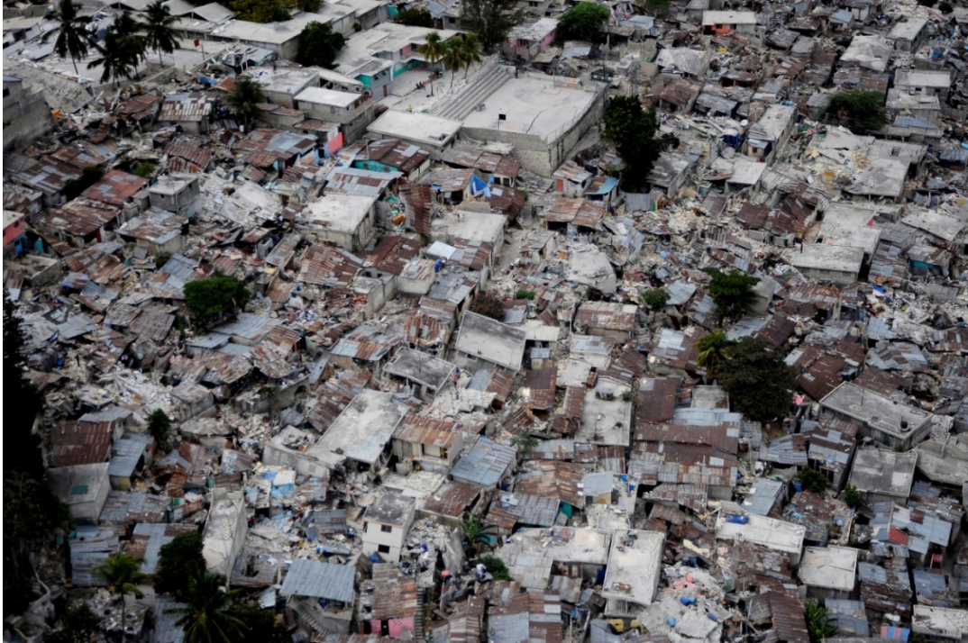
Figure 2.2 Haiti Housing Sector Damage (US Air Force 2011)
