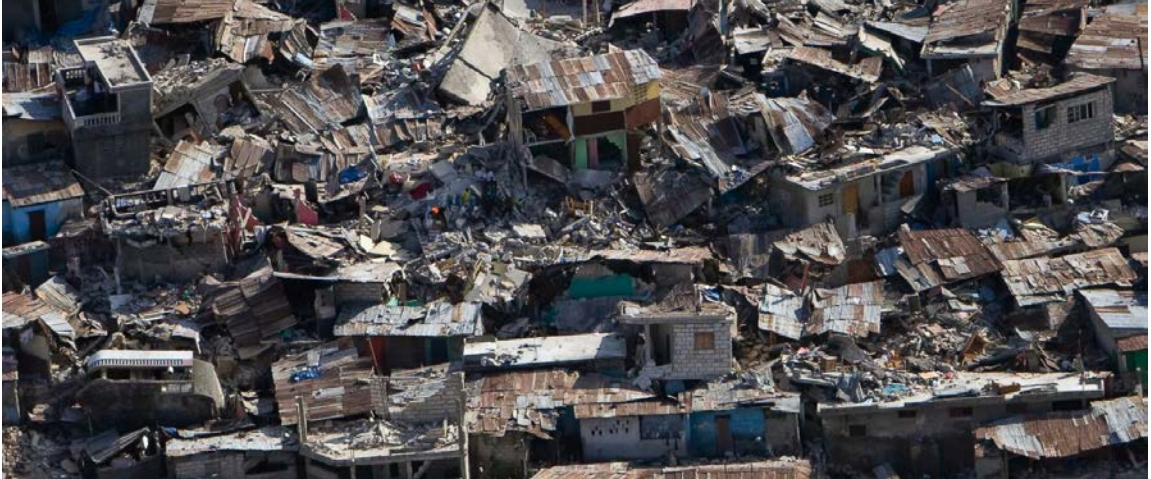
Figure 1.4 – 2010 Haiti earthquake damage (ABC News 2010)
