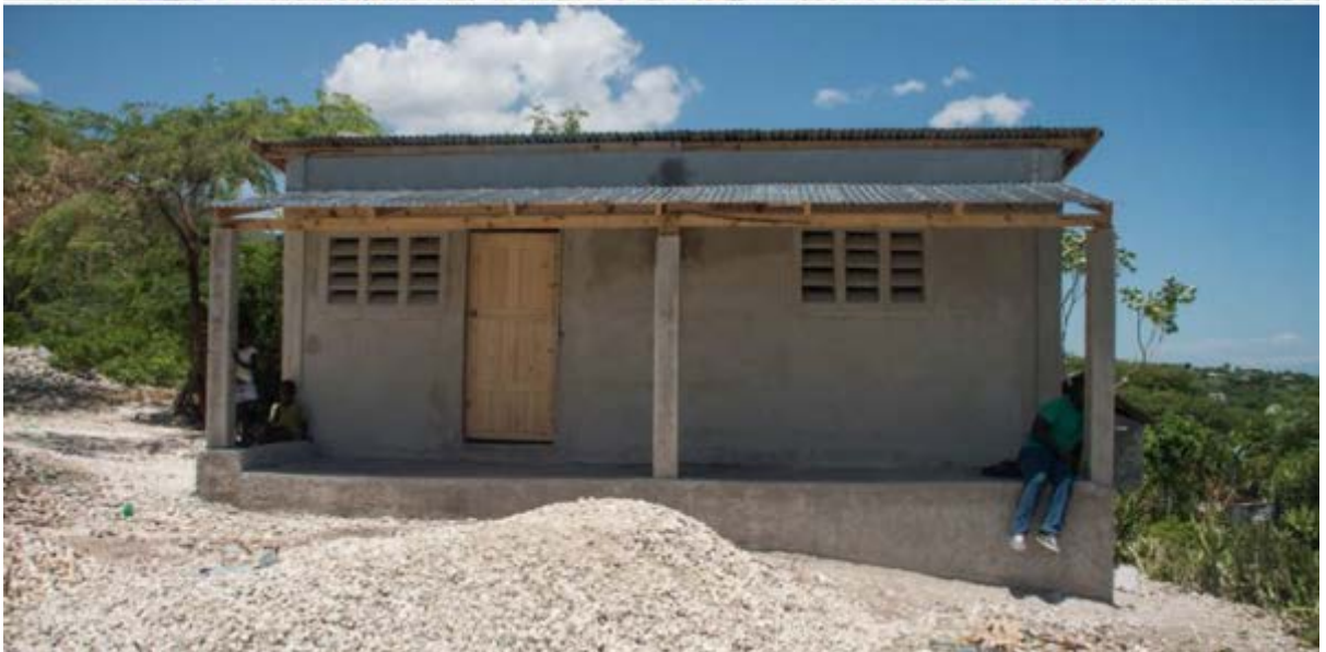
Figure 4.12 Mission of Hope-Haiti housing reconstruction. (MOH-Haiti 2016)
