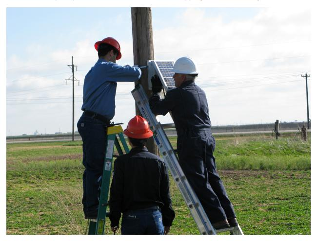
Figure 8.3: Workers installing the sensors on power poles at the Farnsworth, TX site. The nodes, equipped with special mounting brackets, were strapped to the poles with steel strapping. At the request of the site maintainers, great care was taken to not damage the poles.
