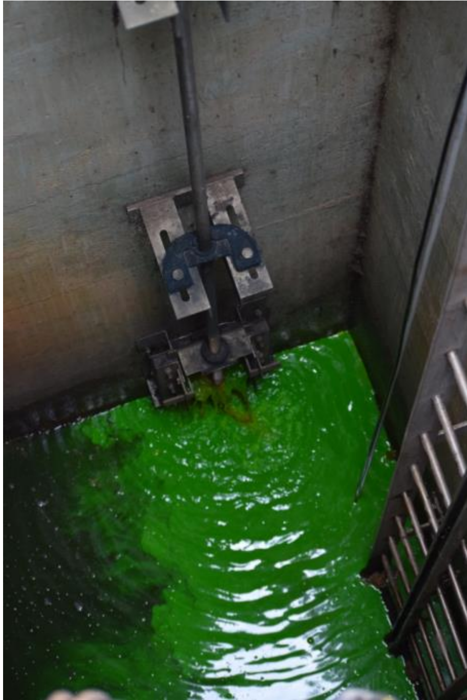
Figure 13. Lift station wet well sewage inflow point during dye test.
