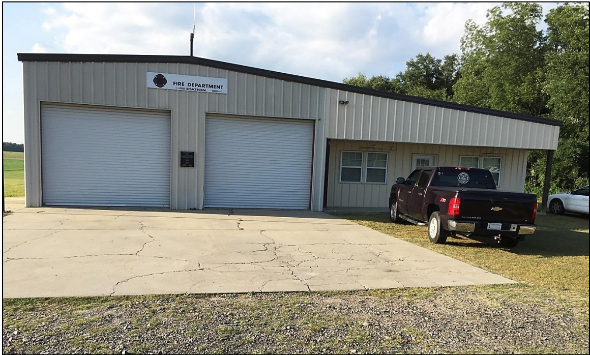
Figure 3-4. A typical fire station in rural South Carolina. (Photo courtesy of Josh Dunn, 2016.)
