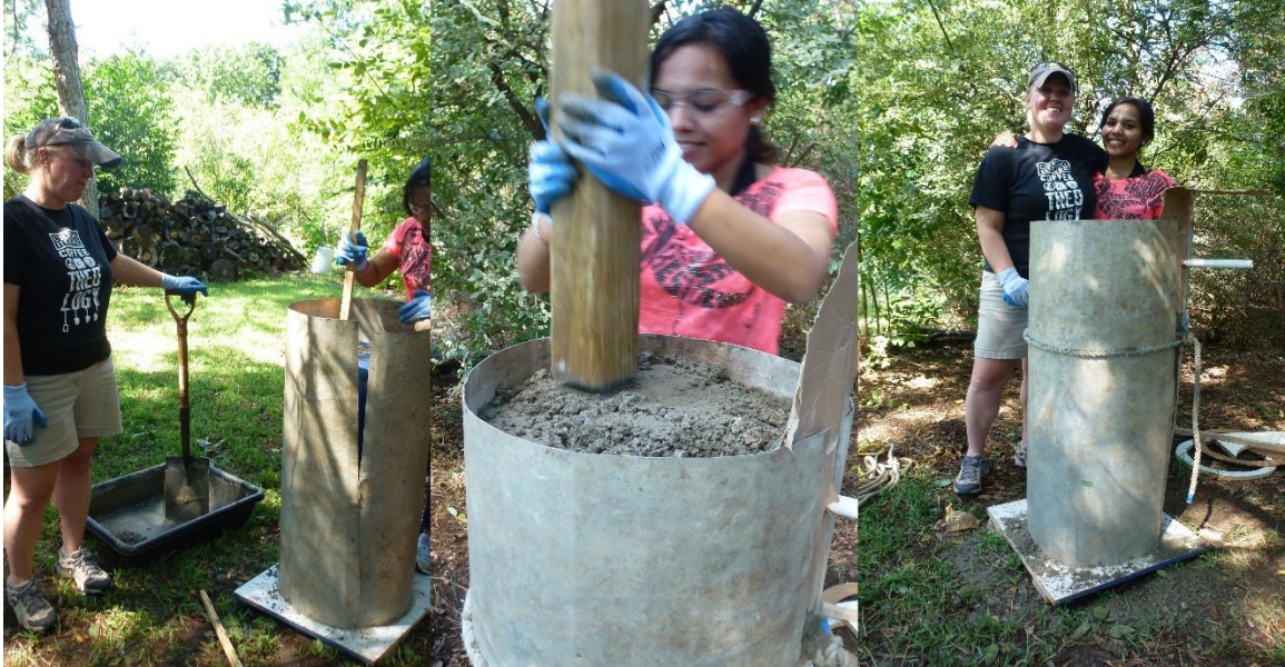
Figure 2. Construction of Bio-Sand Filter using concrete
