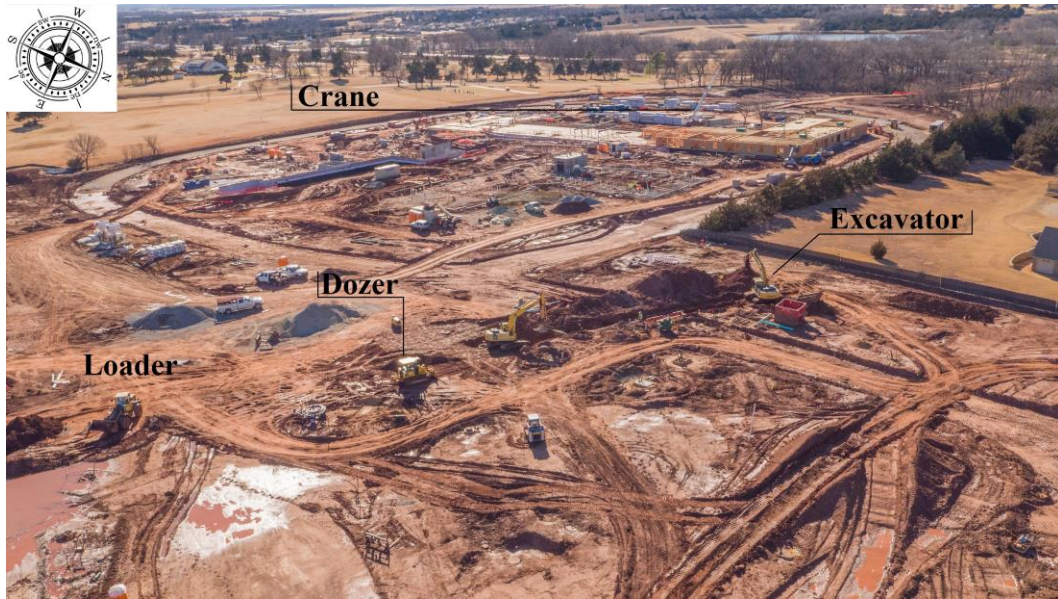
Figure 11: Construction Site and Equipment Fleet
