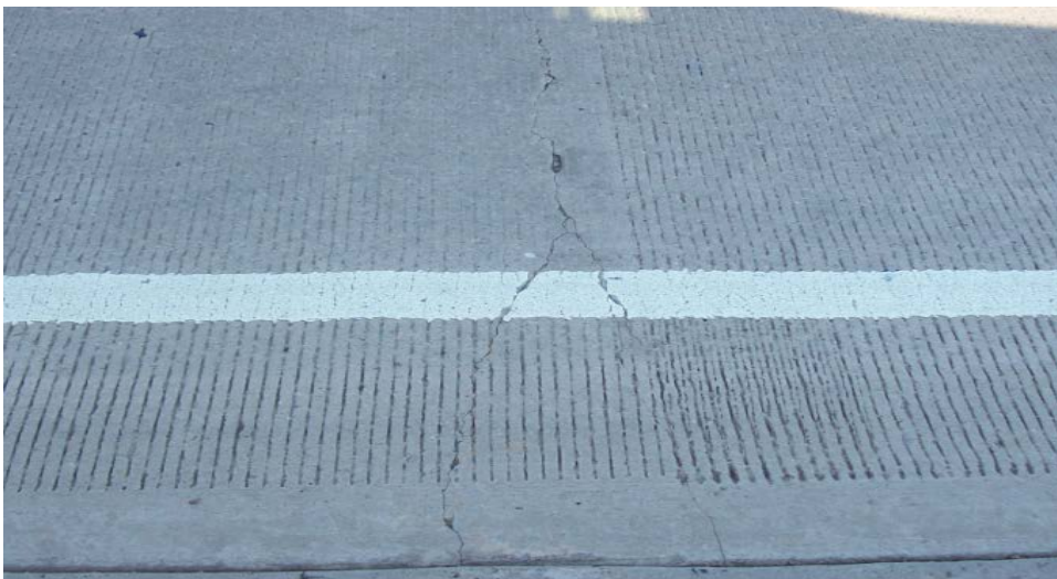
Figure 2.2 Y-cracking example
