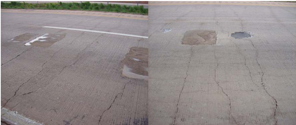
Figure A.82 Roadway patches with exposed steel
