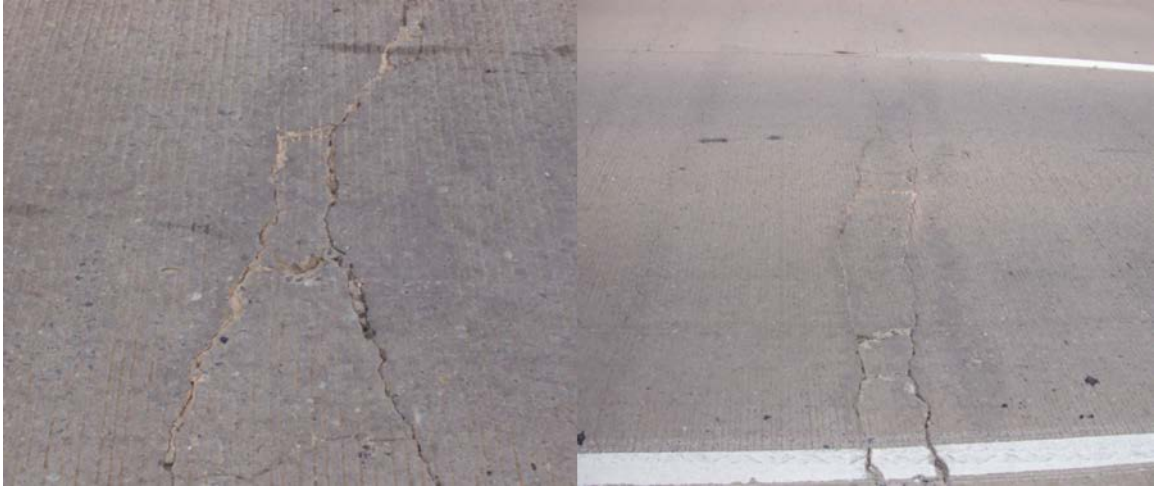
Figure A.54 Two developing punchouts
