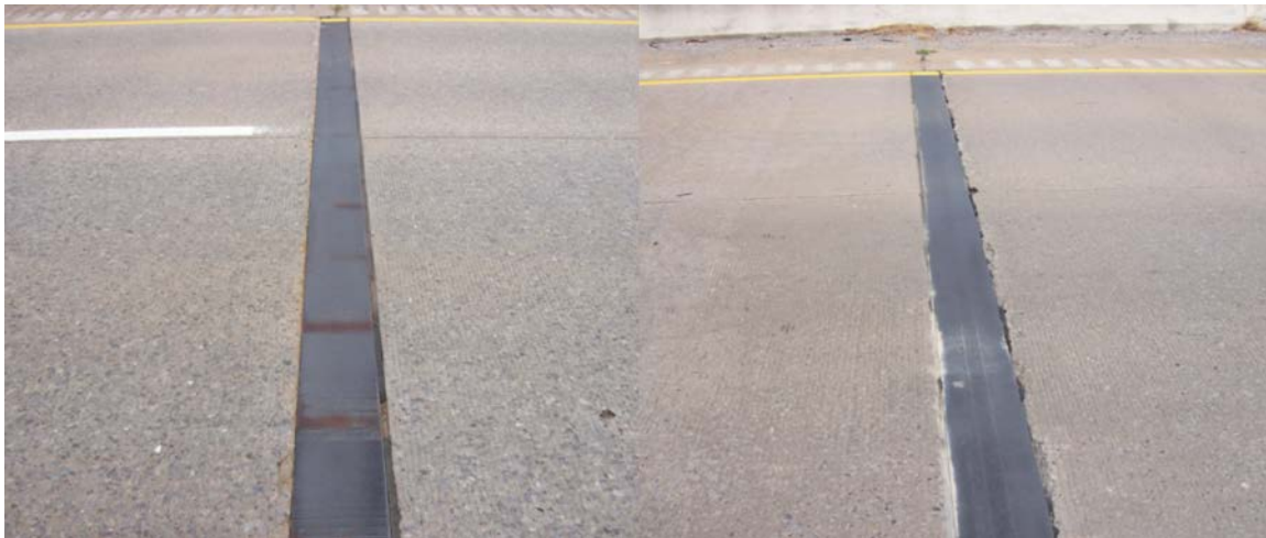
Figure A.61 Terminal joints on each end of the project
