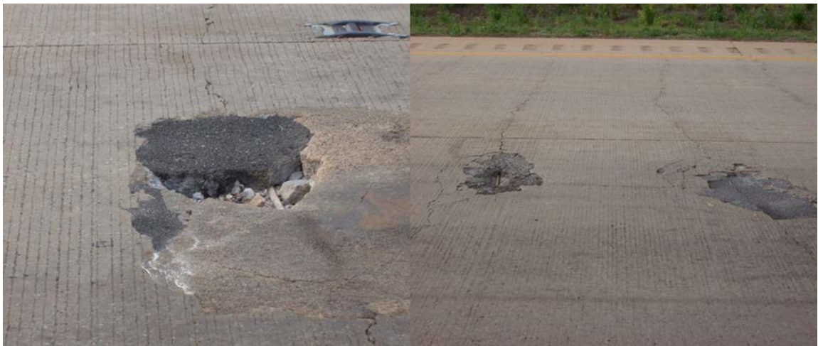
Figure A.82 Roadway patches with exposed steel
