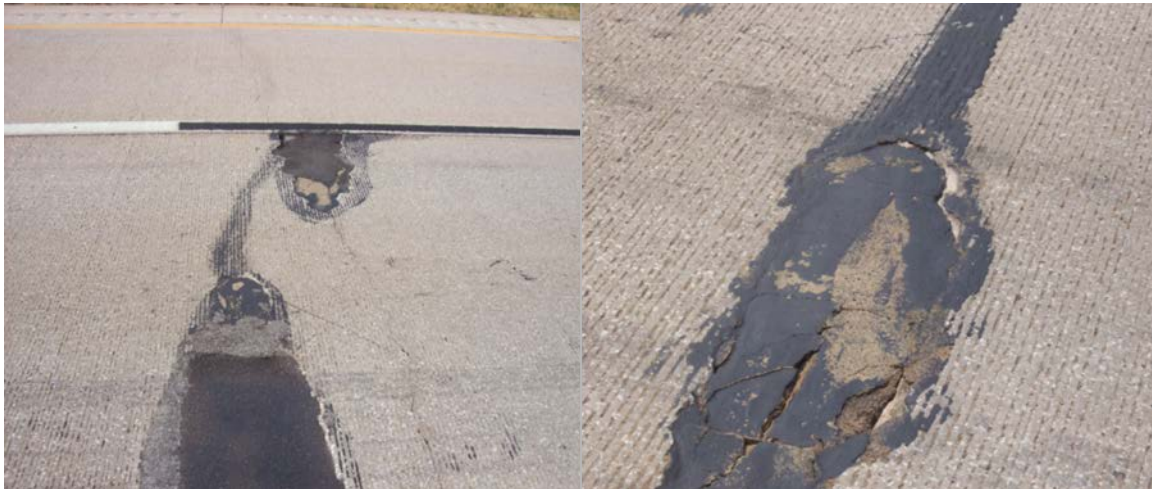
Figure A.27 Y-shaped patches
