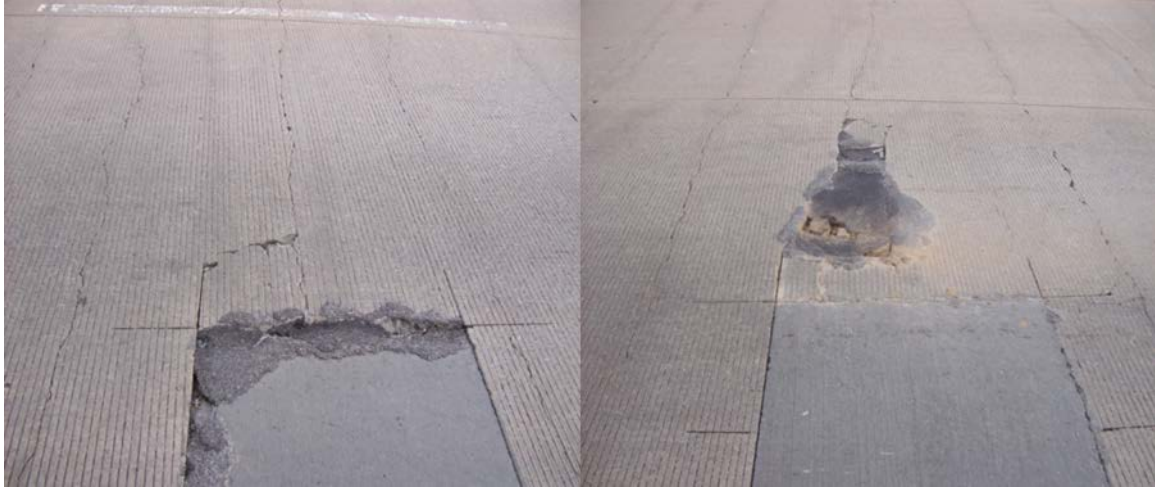
Figure A.32 Small patch with distress developing close by
