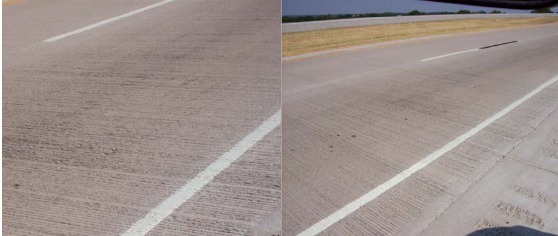
Figure A.18 Two images showing the glossy pavement surface with little wear
