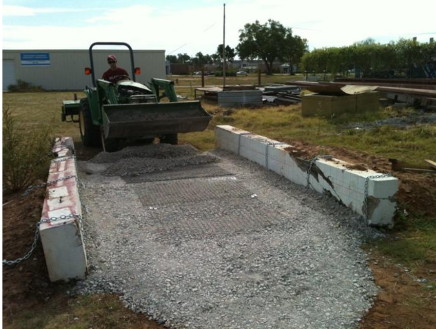
Figure 148. Spreading the second layer of aggregate in the test bed
