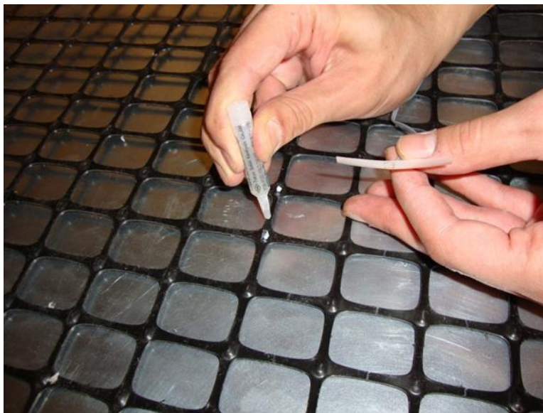
Figure 187. Application of adhesive material to the geogrid
