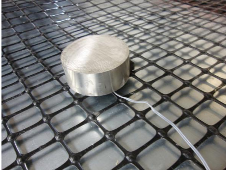
Figure 190. Pressure is applied to the gauge to cure
