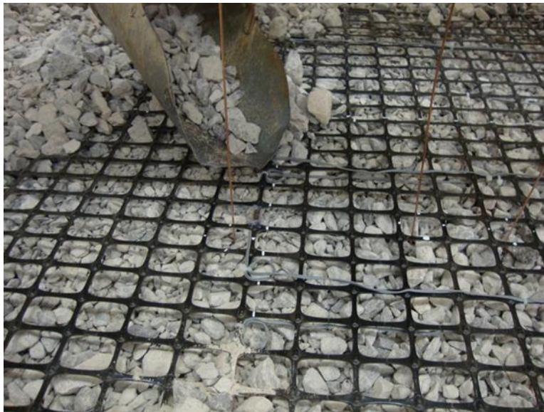
Figure 213. Careful placement of aggregate on the geogrid layer
