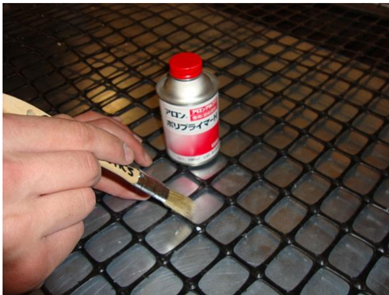
Figure 185. A brush is used to remove dust due to abrasion
