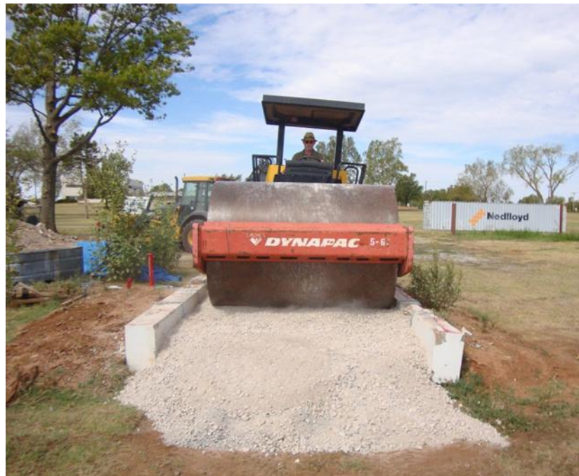
Figure 149. Compacting the second layer of aggregate with the vibratory roller compactor
