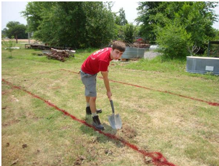
Figure 139. Clearing the test area from existing vegetation
