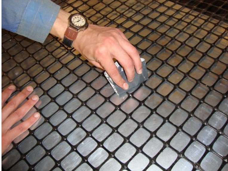
Figure 184. Abrasive paper is used to roughen the surface of the extruded geogrid
