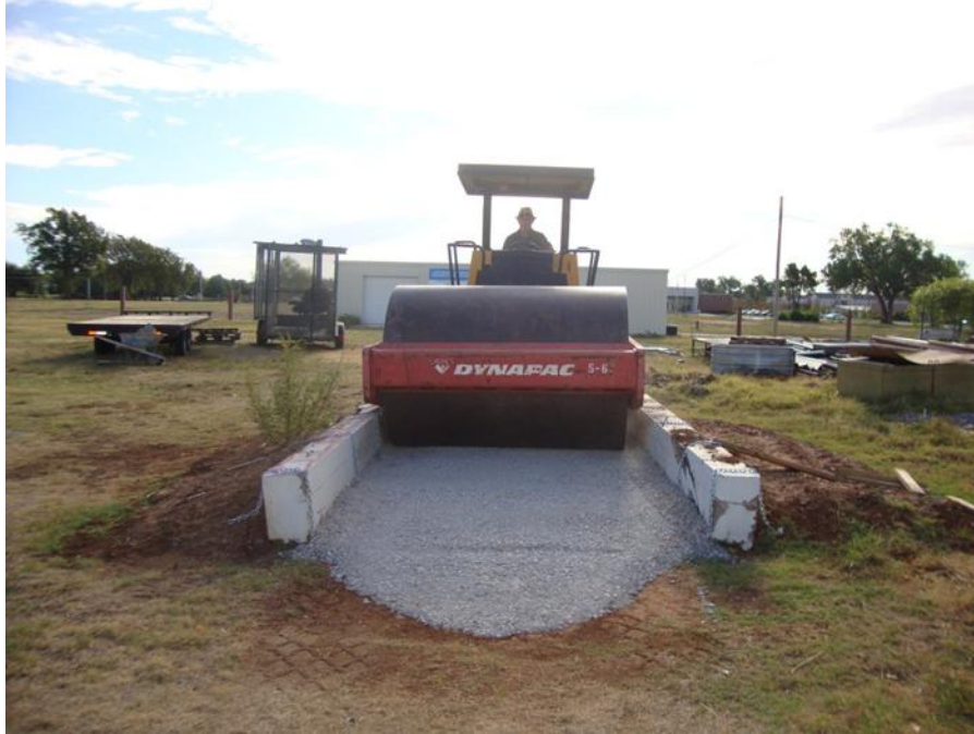
Figure 145. Compacting the first layer of aggregate with a vibratory roller compactor
