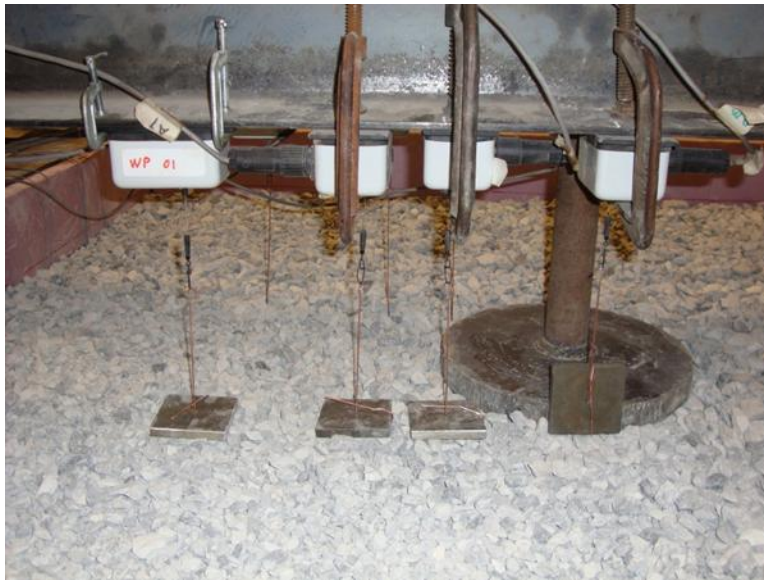
Figure 217. Setup of the wire potentiometers on the top of the aggregate layer
