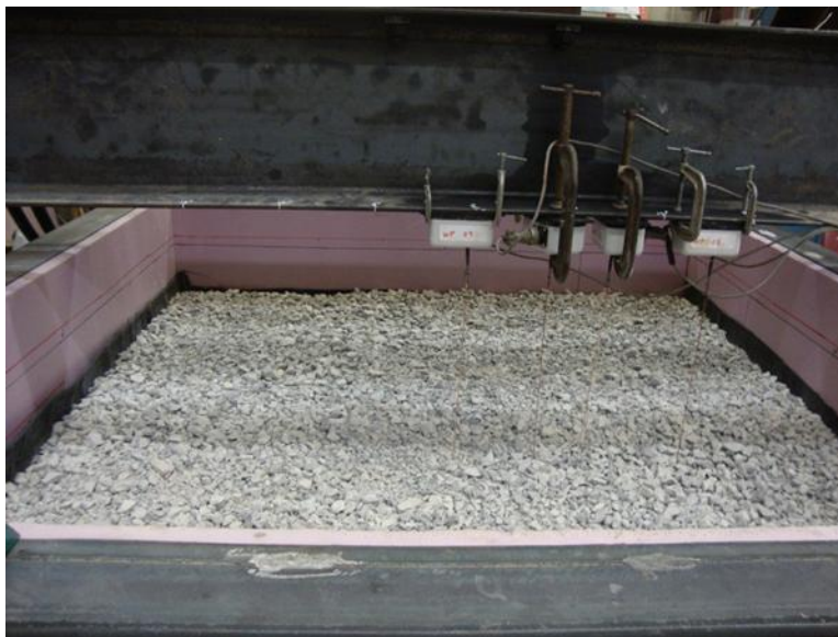
Figure 211. 1-inch-thick aggregate layer placed on the top of the geotextile separator
