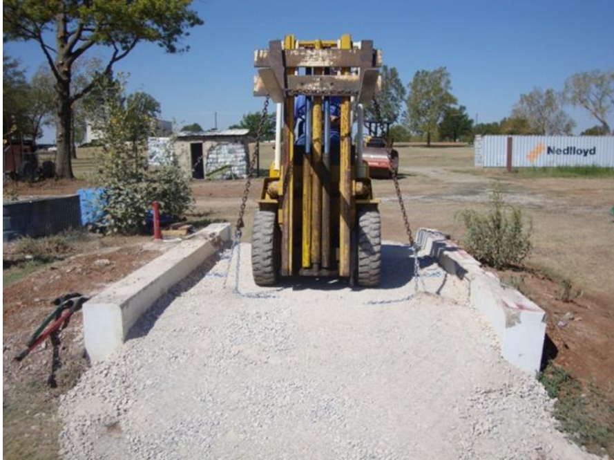
Figure 151. Connecting lifting chains to the forklift
