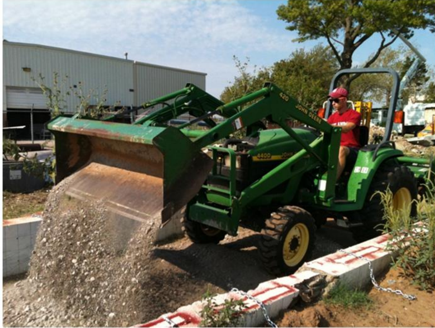
Figure 143. Spreading ODOT Type-A aggregate in the test bed
