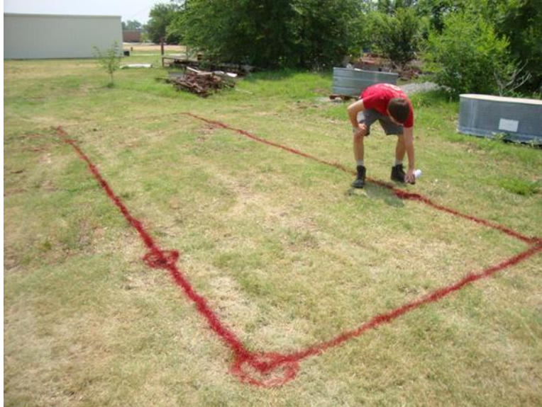
Figure 138. Marking the boundaries of the test site
