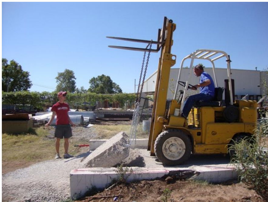
Figure 152. Tilting of steel plates from underneath the compacted aggregate
