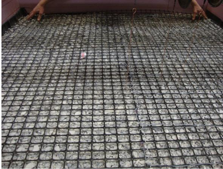
Figure 212. Placing geogrid reinforcement on the 1-inch-thick aggregate layer
