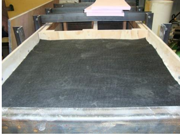
Figure 65. A separator geotextile is placed on the top of the aggregate
