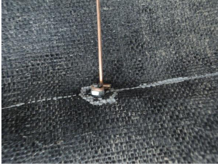
Figure 210. Attachment of brass wires to geotextile separator to measure its settlement
