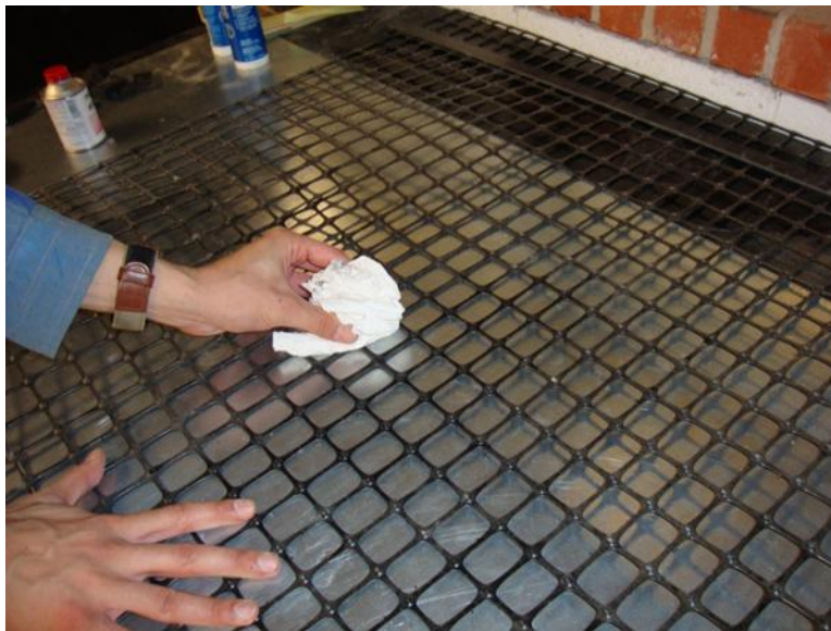
Figure 183. Cleaning the surface of geogrid with industrial tissue or cloth
