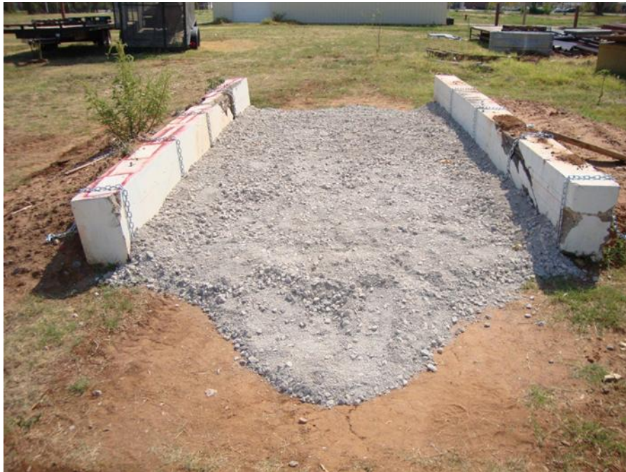
Figure 144. First layer of aggregate in the test bed before compaction
