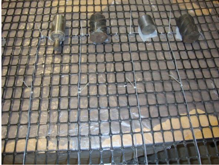
Figure 203. Pressure is applied to the gauges to cure their adhesive layer
