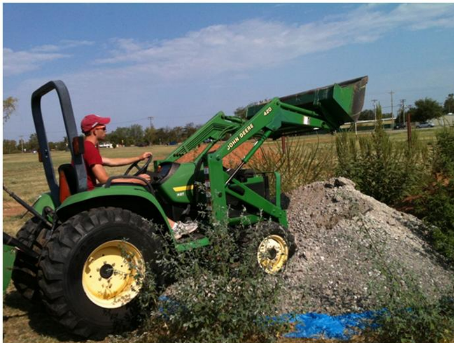
Figure 142. Aggregate was taken from a nearby stockpile using a front-loader tractor
