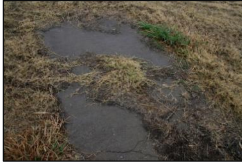
(a) Grass and soil blocks drainage outlets at 19 th St. over I-35
