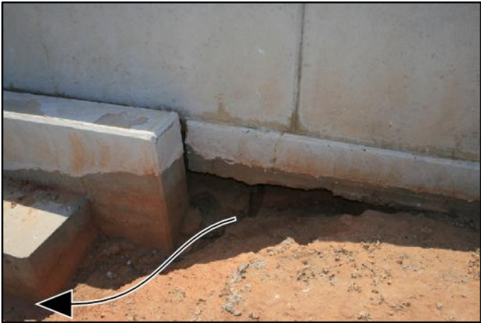
Figure 4.7 Soil flowing laterally from beneath approach slab
