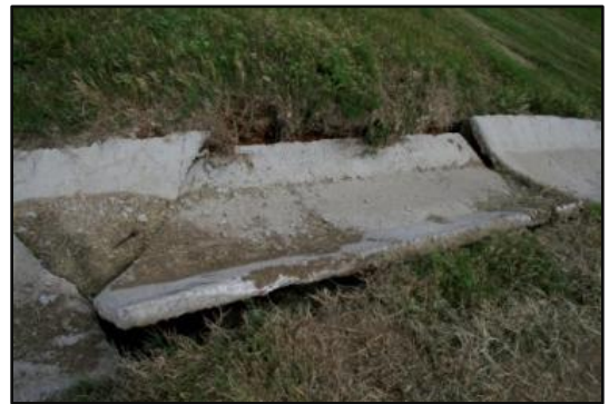
(c) Surface drain channel caving into 3' deep void
