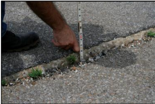
Figure 4.27 Bump at U.S. 177 over Salt Fork, Approach B-2
