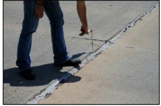
(b) Vertical separation destroys seal
