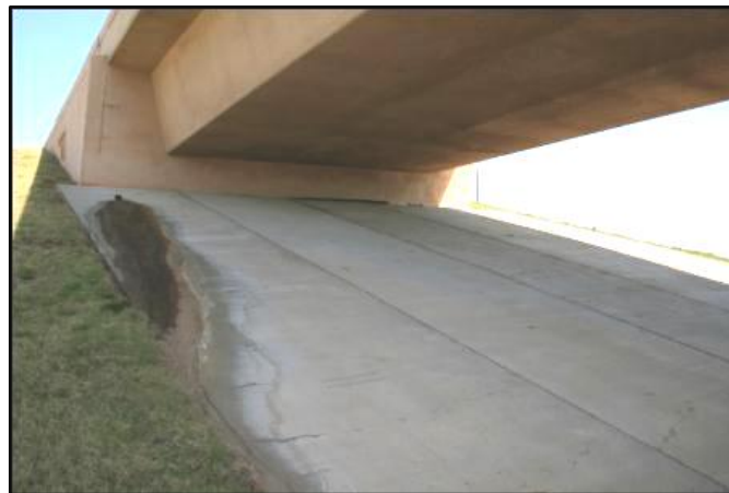
Figure 4.35 Outlet drain at Shields Boulevard over I-35, Embankment N-2
