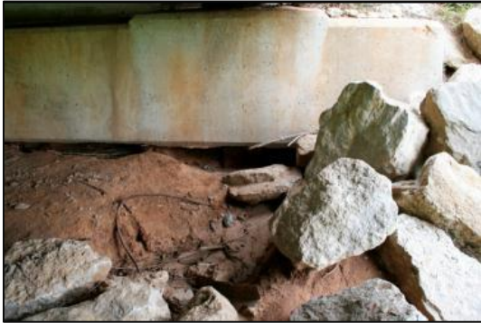
Figure 4.25 Erosion under the abutment on US 177 Embankment A-2
