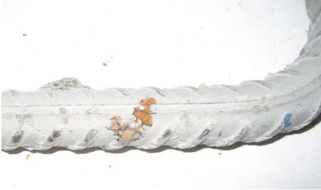
Figure 80a: Corrosion staining on SSClad-b-2 upon autopsy, bent NX-SCR™ stainless steel clad bar (close-up)
