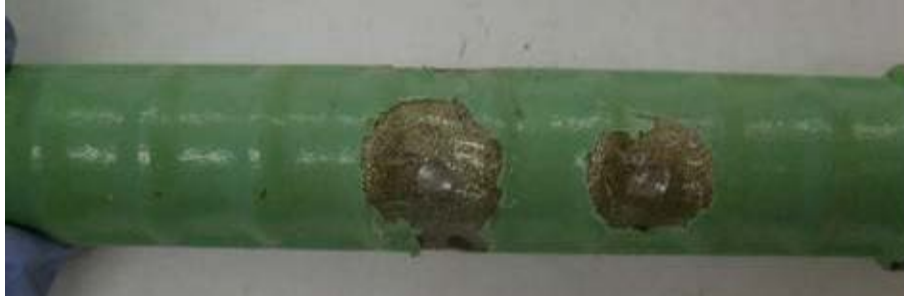
Figure 40: Rapid macrocell specimen upon completion of test, ECR (close-up of damage site after disbondment test)
