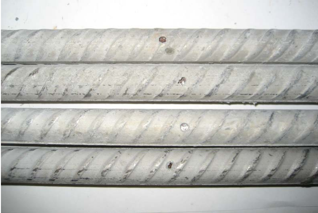
Figure 97c: Bottom bars from Southern Exposure specimen 5 containing stainless steel clad reinforcement with four holes through the cladding after autopsy, showing corrosion at damage site on bottom bars (close up)
