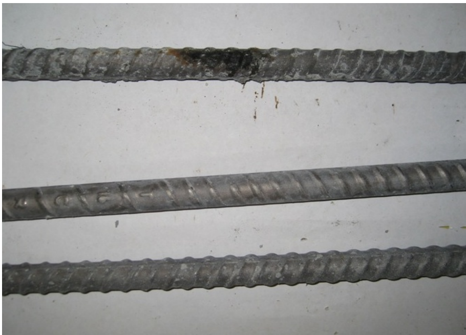
Figure 94a: Bars from cracked beam specimen 1 containing 2304 stainless steel after autopsy
