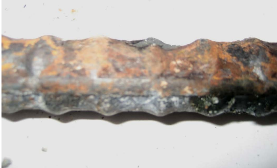
Figure 88c: Close up of conventional top bar in Southern Exposure specimen 3 containing conventional reinforcement as the anode and 2304 stainless steel as the cathode after autopsy
