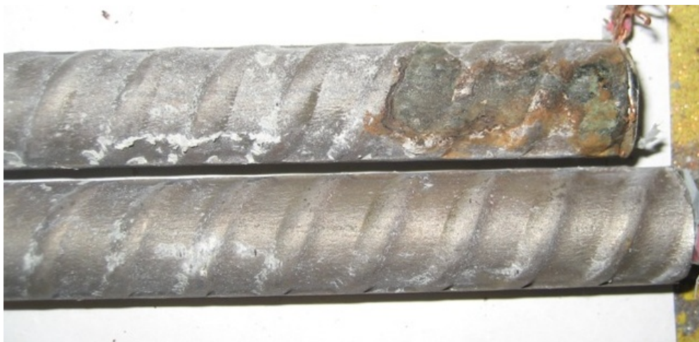
Figure 65a: Top bars of specimen SE-2304-2 after autopsy showing signs of corrosion near the end of the bar
