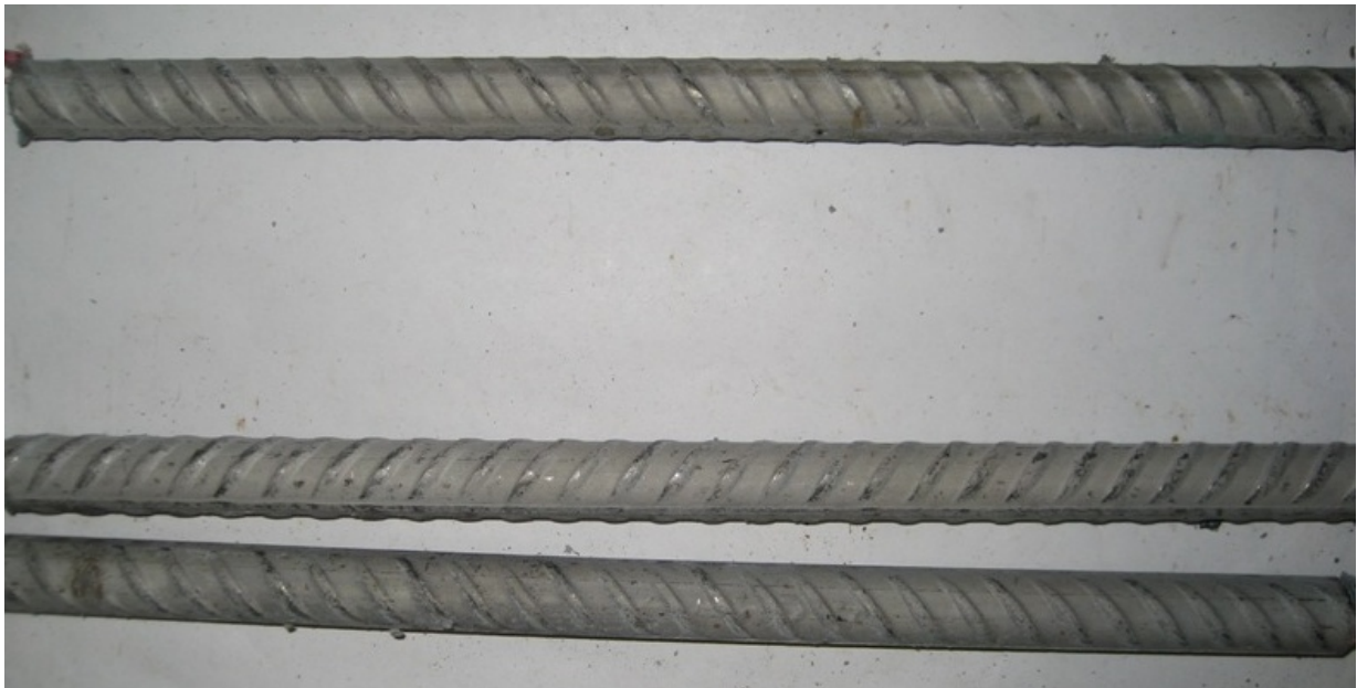
Figure 99: Bars from cracked beam specimen 6 containing undamaged stainless steel clad reinforcement after autopsy
