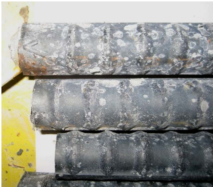
Figure 71: Corrosion on conventional cathode bar in 2304/Conv. Southern Exposure specimen 1 after autopsy
