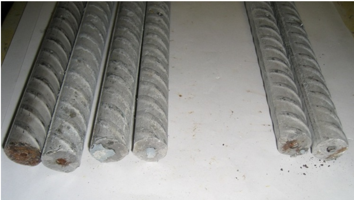
Figure 97d: Bars from Southern Exposure specimen 5 containing stainless steel clad reinforcement with four holes through the cladding after autopsy, showing corrosion at ends of top and bottom bars (close up)
