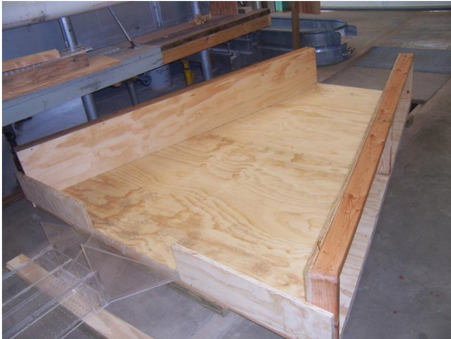
Figure 9. Downstream plywood channel after wingwall
