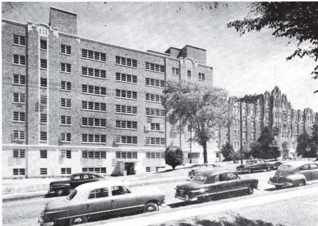
Pictured above is the attractive new eight-story addition to Hillcrest Memorial Hospital, 1653 East 12th, Tulsa, as it neared completion. To the right is the original structure which now joins the new wing. (Photo by Hopkins).
