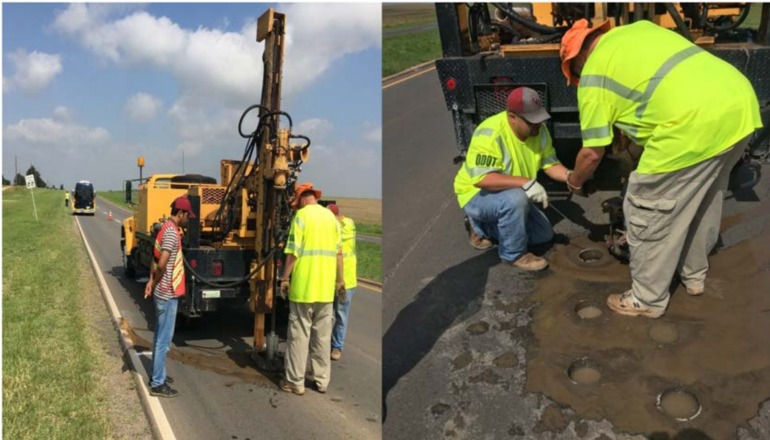
Figure 72. Collection of the Field Cores from the Construction Site
