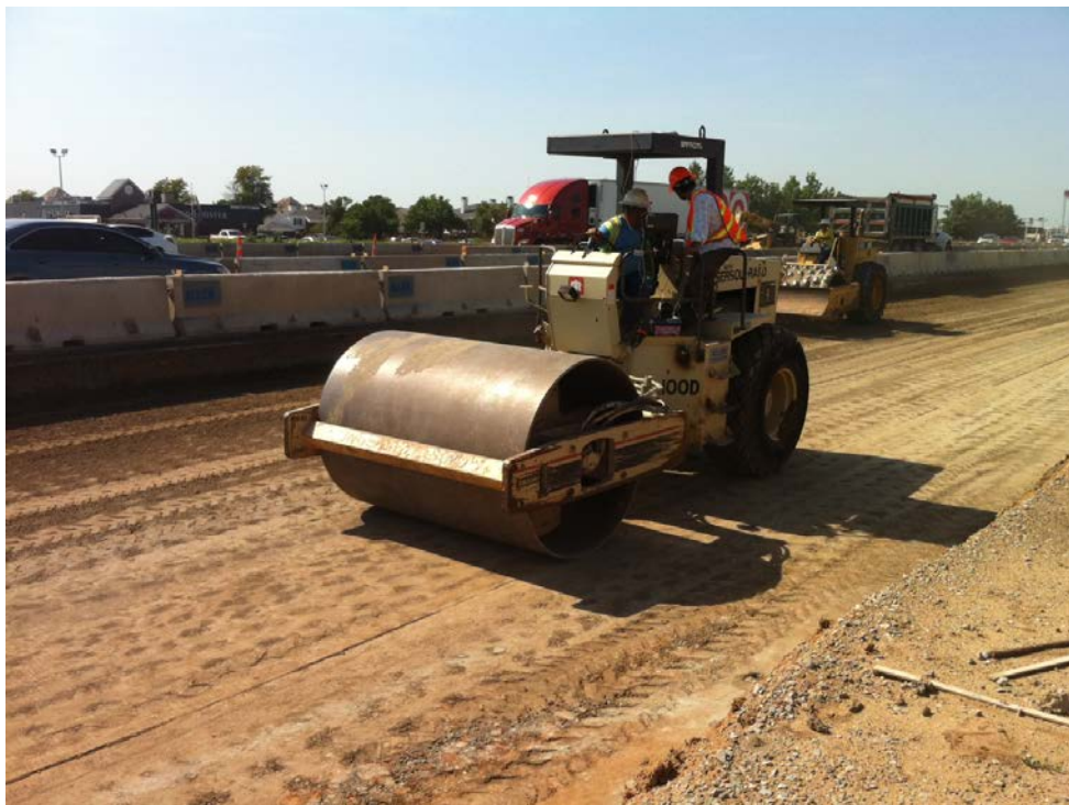
Figure 5.6. ICA compaction in progress.
