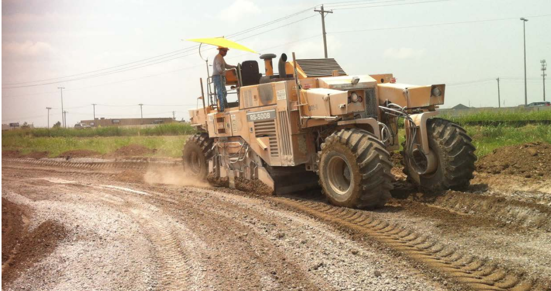
Figure 6.4. Pre-treatment of existing soil by 3% lime at the I-35 Service Road Project.
