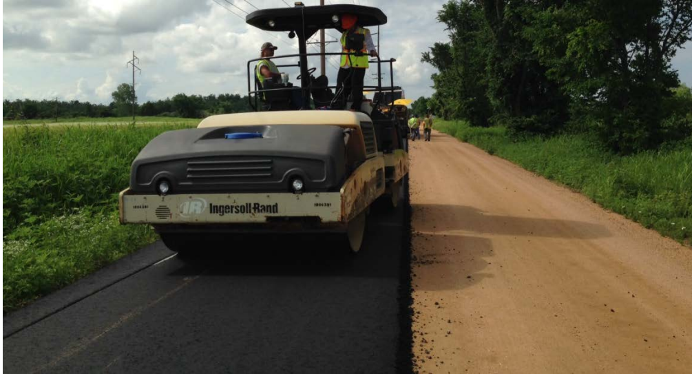
Figure 9.5. Recording ICA measurements during the compaction of the base layer.
