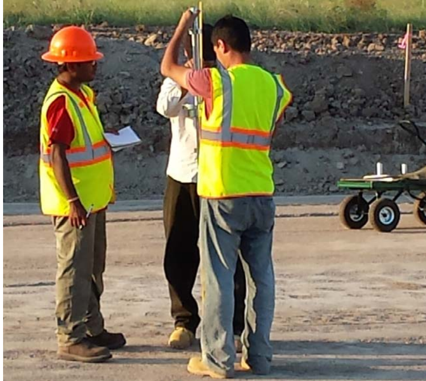
Figure 6.15. DCP test on the compacted subgrade at the I-35 Service Road project.
