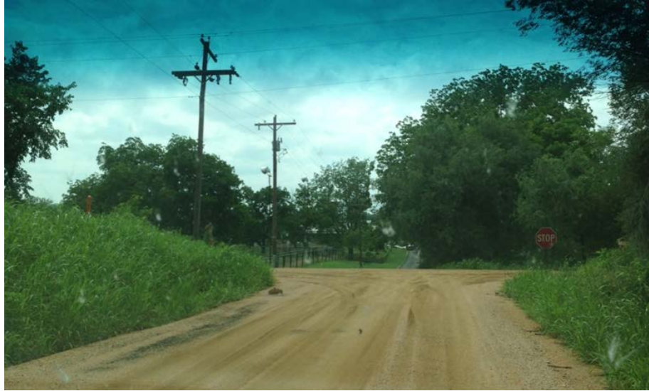
Figure 9.2. Unstabilized granular layer to support the asphalt base layer.
