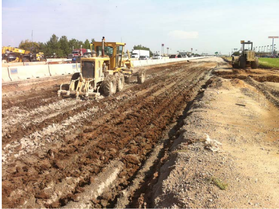
Figure 5.2. Mixing of CKD with soil at the I-35 project in Norman, OK.
