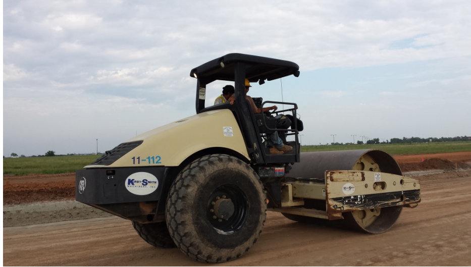
Figure 6.9. ICA compaction of soil-lime-CKD mix with smooth drum vibratory roller at the I-35 Service Road project.
