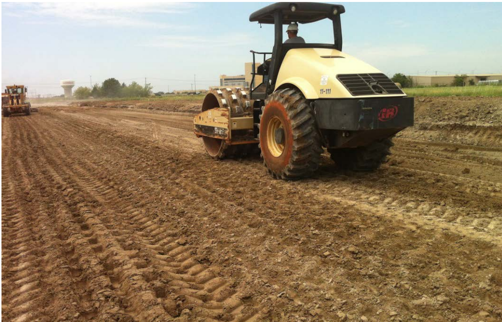
Figure 6.8. Initial compaction of soil-lime-CKD mix with pad-foot roller at the I-35 Service Road project.
