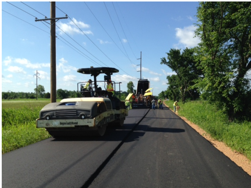
Figure 9.6. Recording ICA measurements during the compaction of the surface layer.
