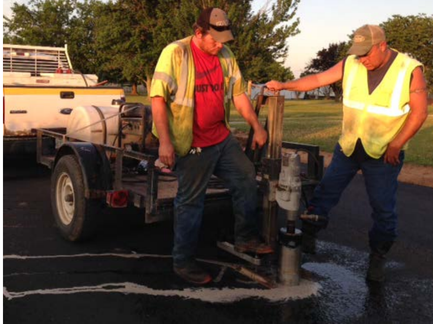
Figure 9.4. Extraction of roadway cores from Acme Road project.
