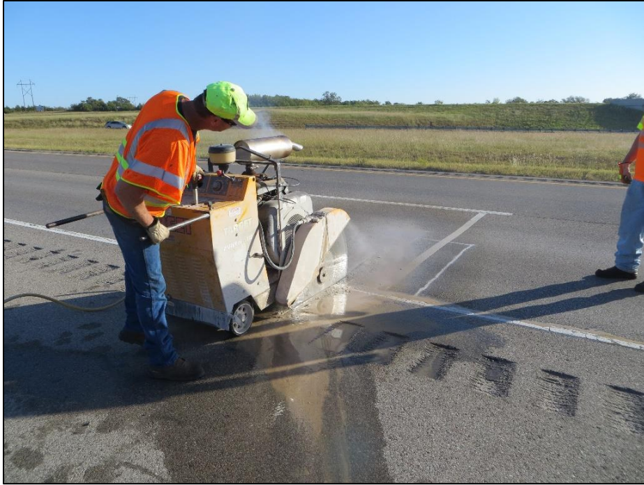
Figure 19: Cutting of Trench using Saw-cutting Machine
