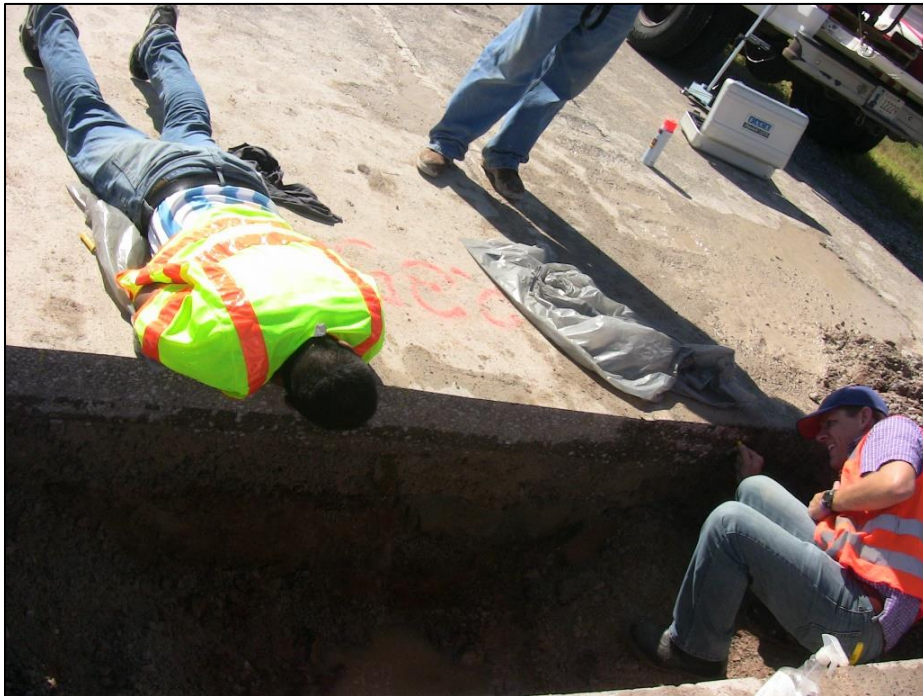
Figure 22: Marking of Different Pavement Layers
