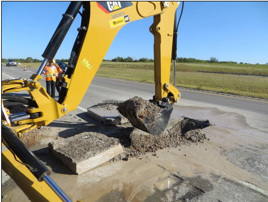
Figure 20: Removal of Pavement Materials using Back-hoe
