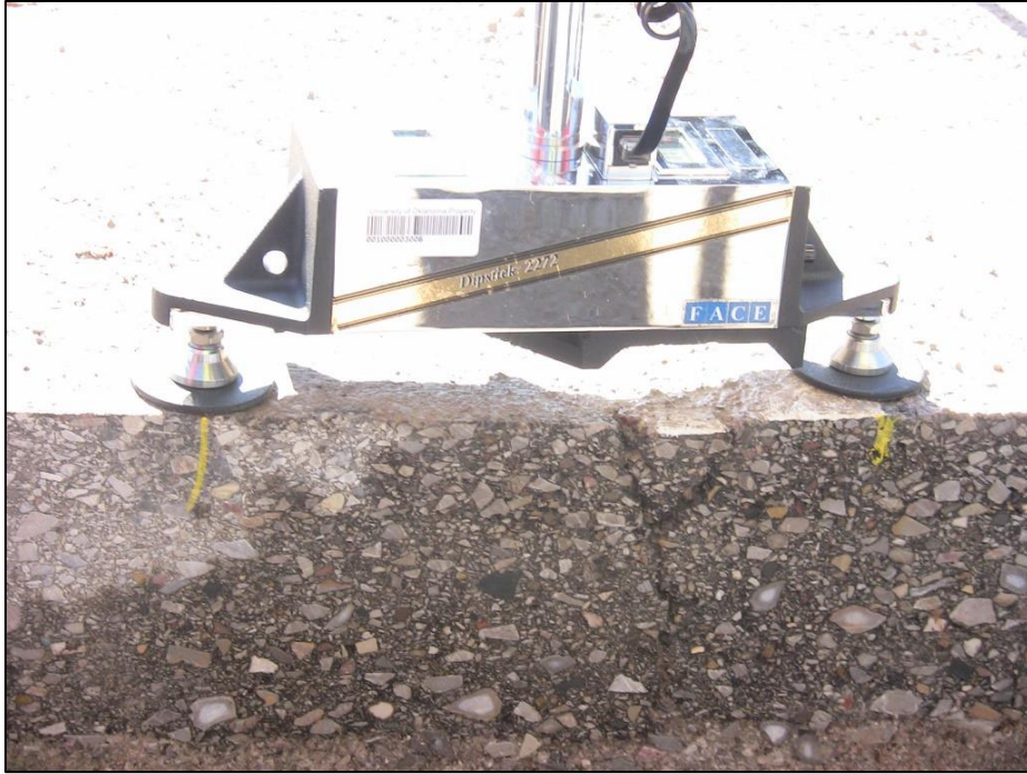
Figure 21: Rut Measurements using Face Dipstick®
