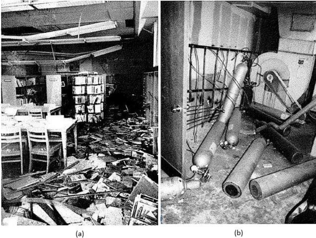
Figure 1.1: Examples of nonstructural damage: (a) toppling book cases and (b) damage to gas canisters. Source: McKeivitt et al. (1995).
