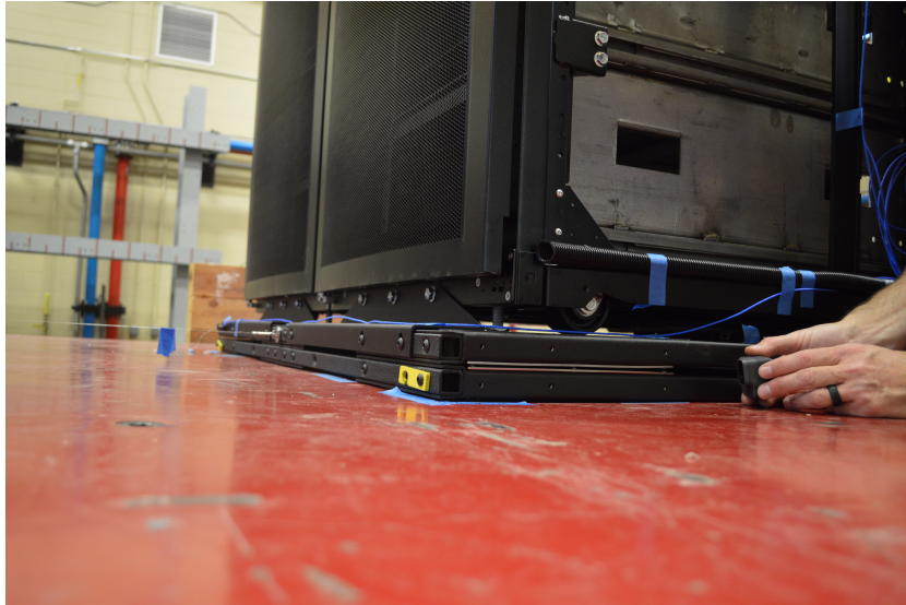
Figure 3.13: Reduced platform clearance of isolation system.
