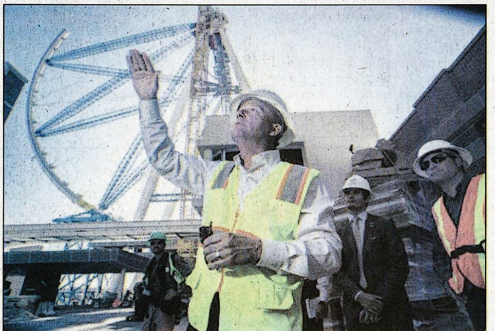
In a Tuesday, July 30, 2013 file photo, the world's tallest observation wheel, known as the High Roller is seen behind David Codiga, executive project director for The Linq, at The Linq construction site on Las Vegas Boulevard. The outer wheel of the 55-story High Roller ride is scheduled to be hoisted into place Monday, Sept. 9, 2013. (AP Photo/Las Vegas Review-Journal, Jeff Scheid, File)
