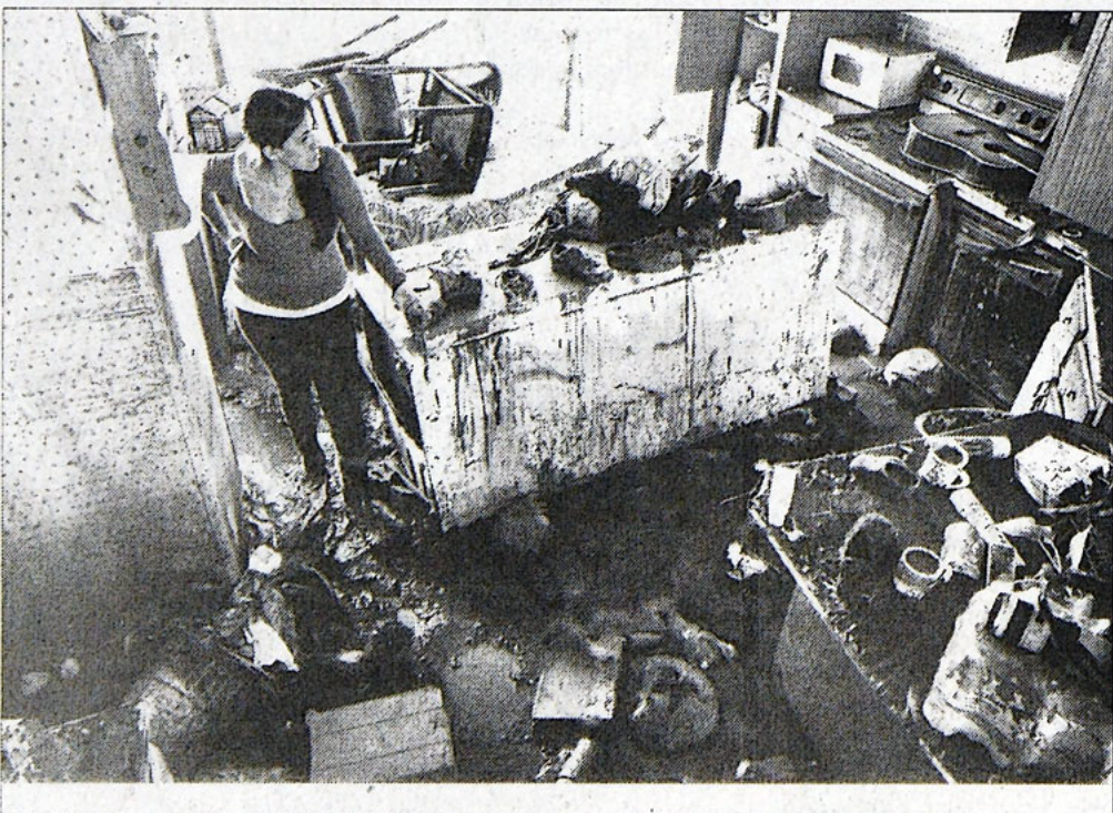
In this Sept. 24, 2013 photo, Sonia Marquez, an organizer with the Colorado Immigrant Rights Coalition, looks for keepsakes amid the muck inside one of the many homes now declared uninhabitable due to permanent flood damage at a decimated trailer park in Evans, Colo. The majority of the residents in the trailer park are immigrants who didn't have flood insurance, and because some are not citizens or legal residents, they can't get government help. (AP Photo/Brennan Linsley)
