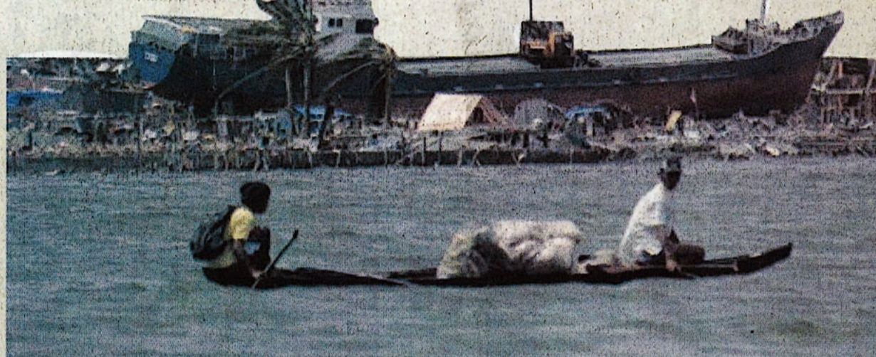
A ship that was washed ashore lies under damaged houses in Tacloban city, Leyte province, central Philippines on Monday, Nov. 11, 2013. Typhoon Haiyan-ravaged Philippine islands faced a daunting relief effort that had barely begun Monday, as bloated bodies lay uncollected and uncounted in the streets and survivors pleaded for food, water and medicine. (AP Photo/Aaron Favila)
