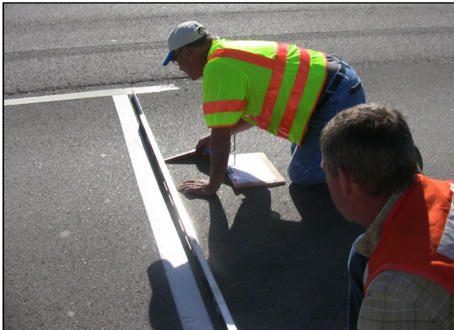
Figure 3.8: Rut Measurements with Straight Edge/Rut Gauge Combination (Hossain et al., 2010)
