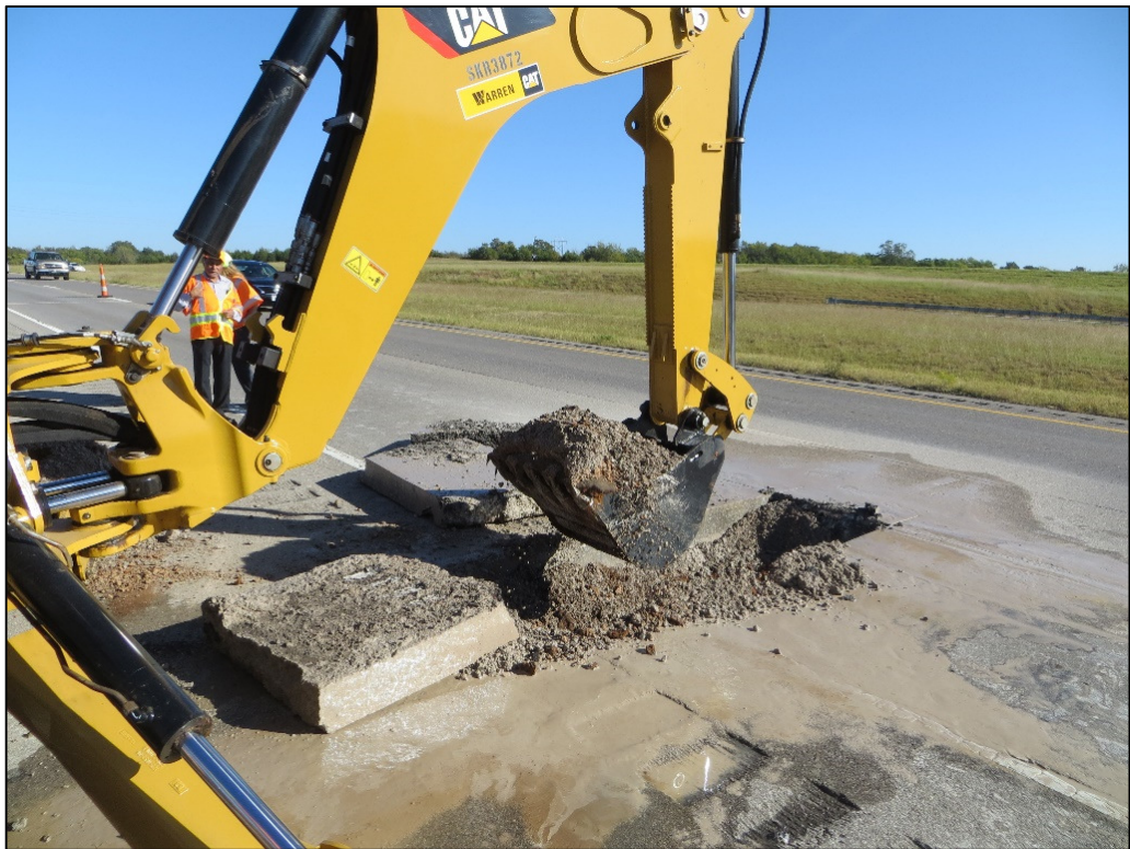
Figure 7.8: Removal of Pavement Materials using Back-Hoe
