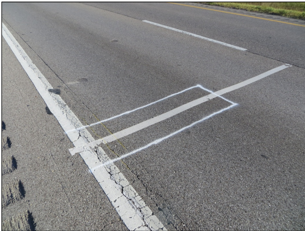
Figure 7.6: Marking on the Test Section before Trenching Operations
