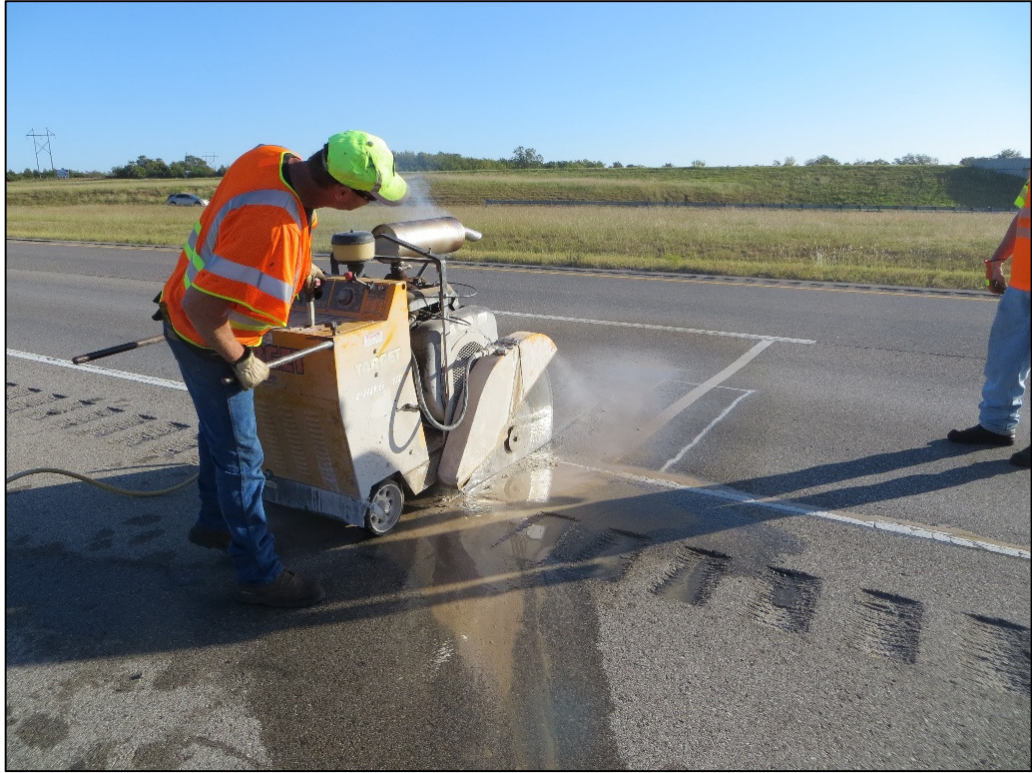
Figure 7.7: Cutting of Trench using Saw-cutting Machine
