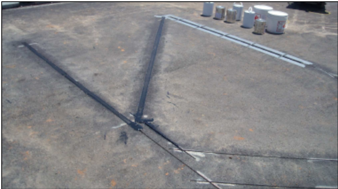
Figure 3.5: Dynax® Lateral Positioning Sensors (Solanki et al., 2013)
