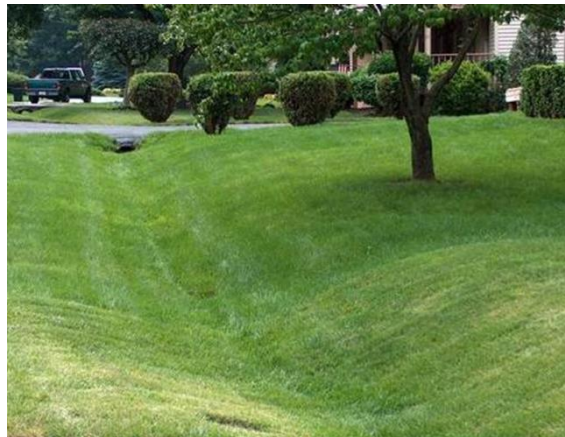
Figure H-1. Grass-lined channel illustration (Virginia DEQ, 2014)
