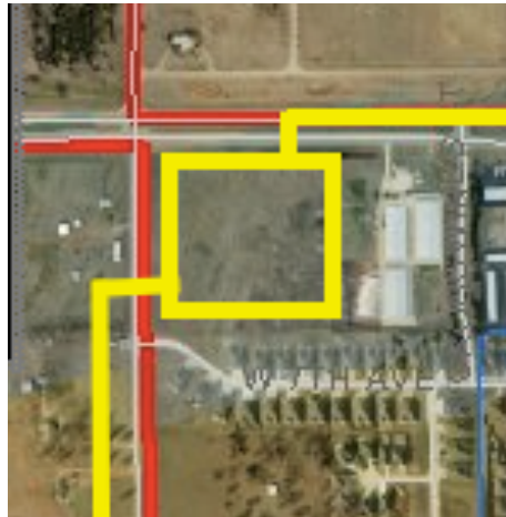
Figure 4.1-1: Booster station location. The red lines are Stillwater city limits, and the yellow square is the site of the station. Range Road runs along the west side of the station, and Highway 51 runs along the north side.
