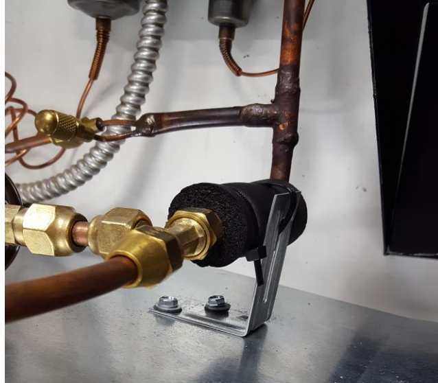
Figure 17: Copper tubing support installed
