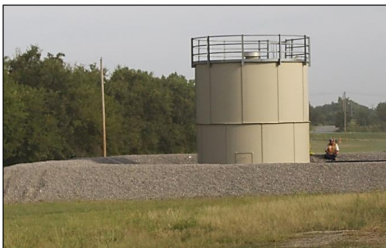
Figure 28: Enid Municipal Landfill leachate collection tank
