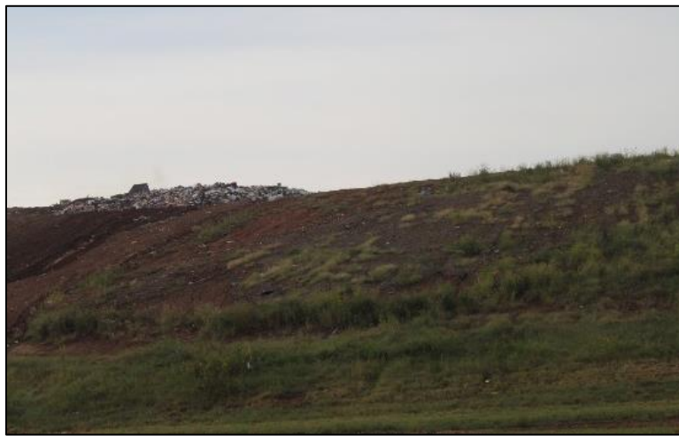
Figure 21: Current mulch use existing at the Enid Municipal Landfill
