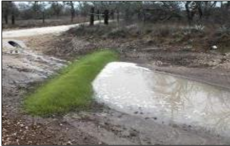
Figure 45: Example of compost berm implementation (EPA)
