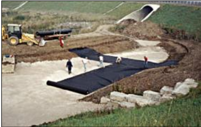
Figure 10: Nonwoven textile fabric application (Layfield Construction Products)
