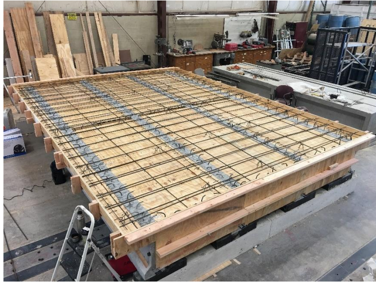
Figure 68: Scale bridge formwork showing steel in both directions
