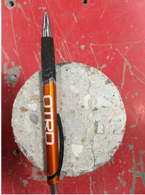
Figure 31: Crack on web core W3
