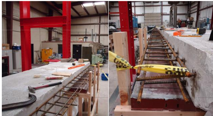
Figure 20: Construction of deck extension of girder C in progress
