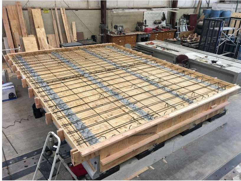
Figure 73: Bridge section with reinforcing steel
