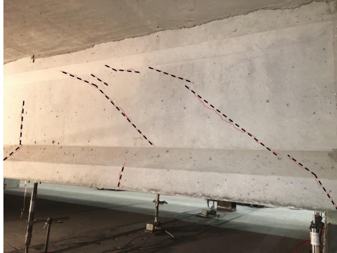
Figure 101: Cracking at 67 kips of load for the loaded girder
