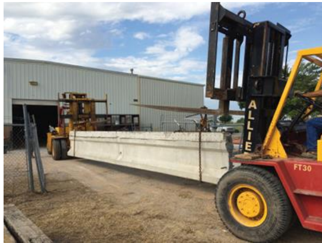
Figure 16: Transportation of girder A into Fears Lab on July 29, 2014
