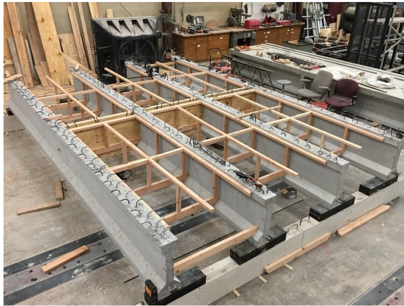
Figure 71: Framing for bridge deck formwork including middle diaphragm
