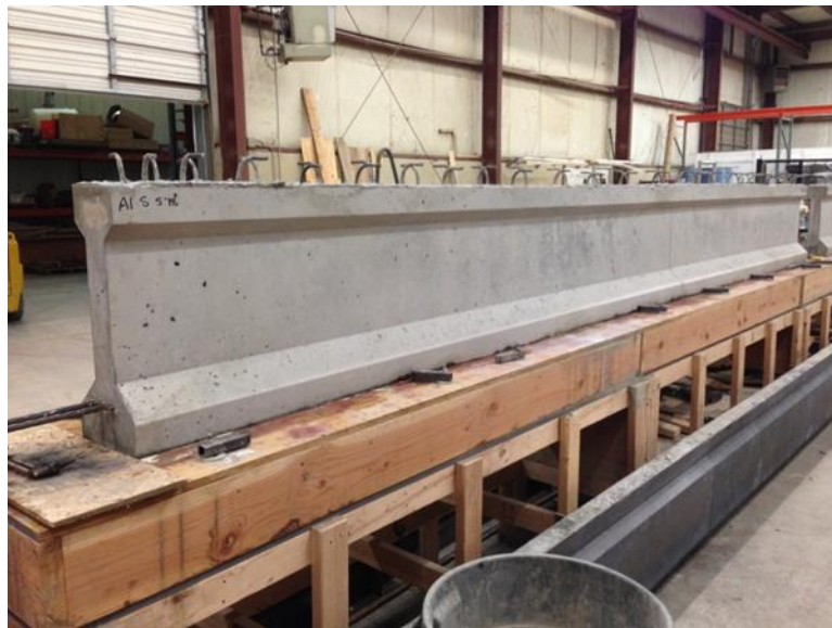
Figure 63: Completed scale girder before cutting prestressing strands
