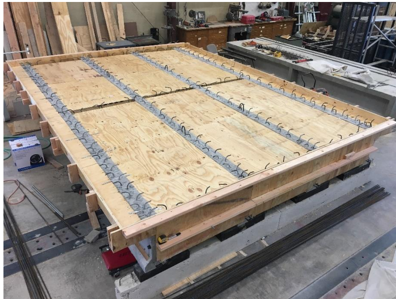
Figure 72: Completed deck formwork showing end diaphragms and edges of deck
