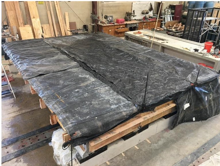
Figure 78: Plastic covering wet burlap laid on the bridge deck while curing
