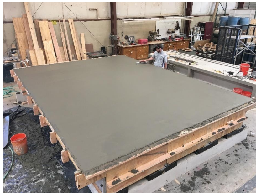
Figure 76: Bridge after screeding and floating
