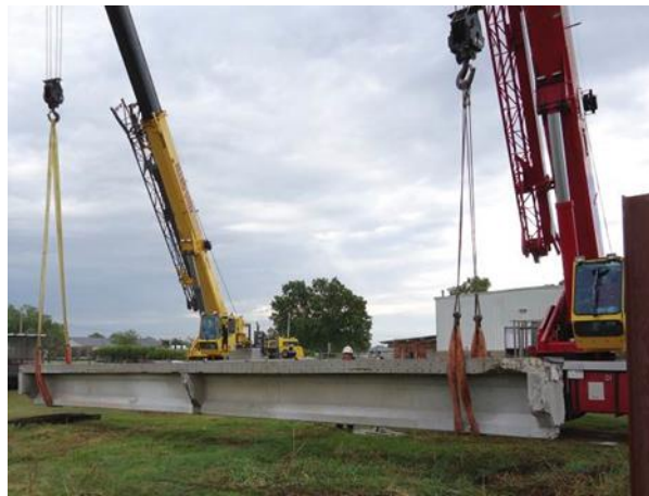
Figure 13: Unloading of girder C using 20 ton rental cranes on October 8, 2013
