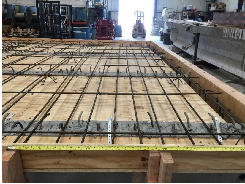
Figure 74: Close up of deck reinforcement including rebar chairs
