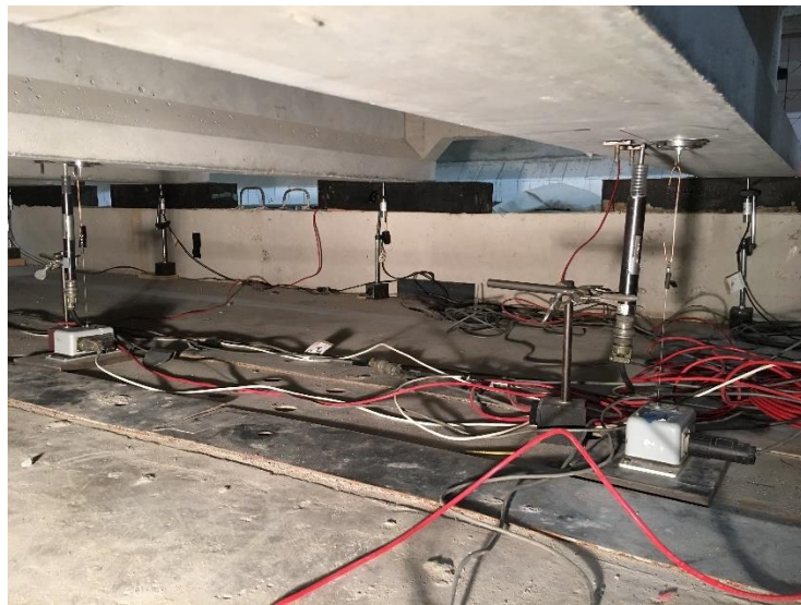
Figure 83: Underside of girders prior to destructive test showing LVDTs and wire pots used to measure deflection as well as LVDTs at the supports in the background
