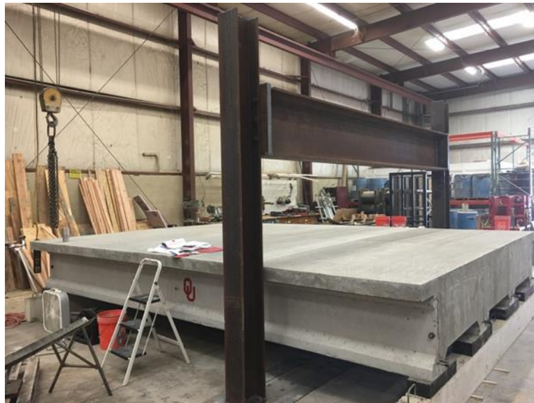
Figure 79: Load frame as installed over bridge and completed bridge after curing
