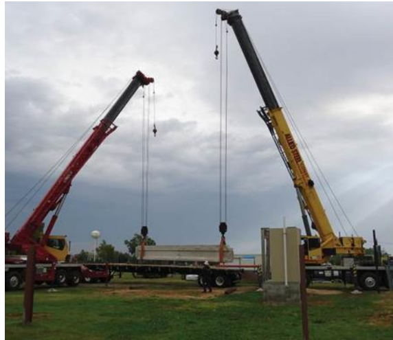
Figure 12: Unloading of girder A using 20 ton rental cranes on October 8, 2013
