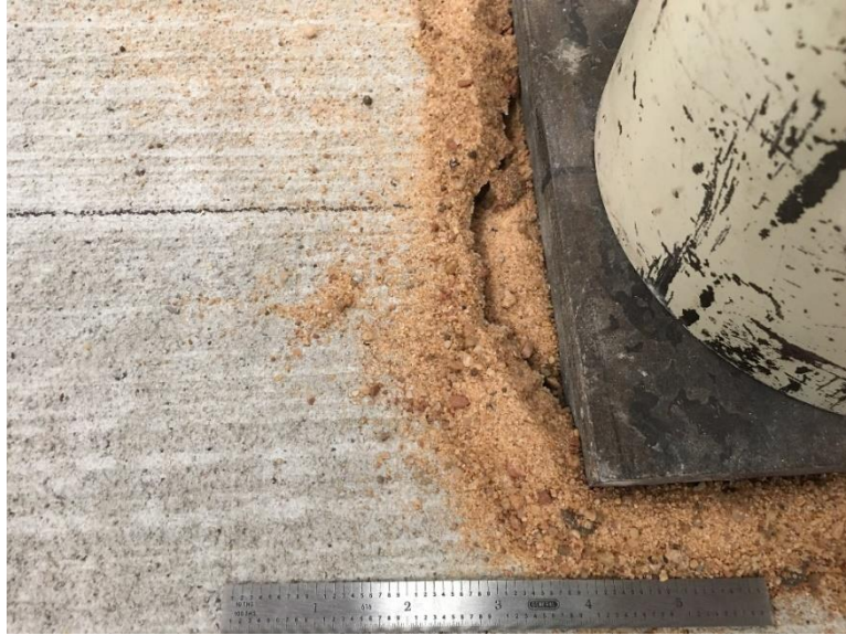
Figure 105: Punching shear failure in slab at load point
