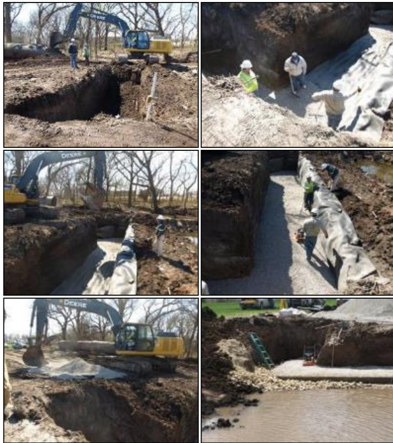
Figure 75: A GRS-IBS (Bridge No. 3) under construction near Blackwell in Kay County with sheet piling for the abutment facing
