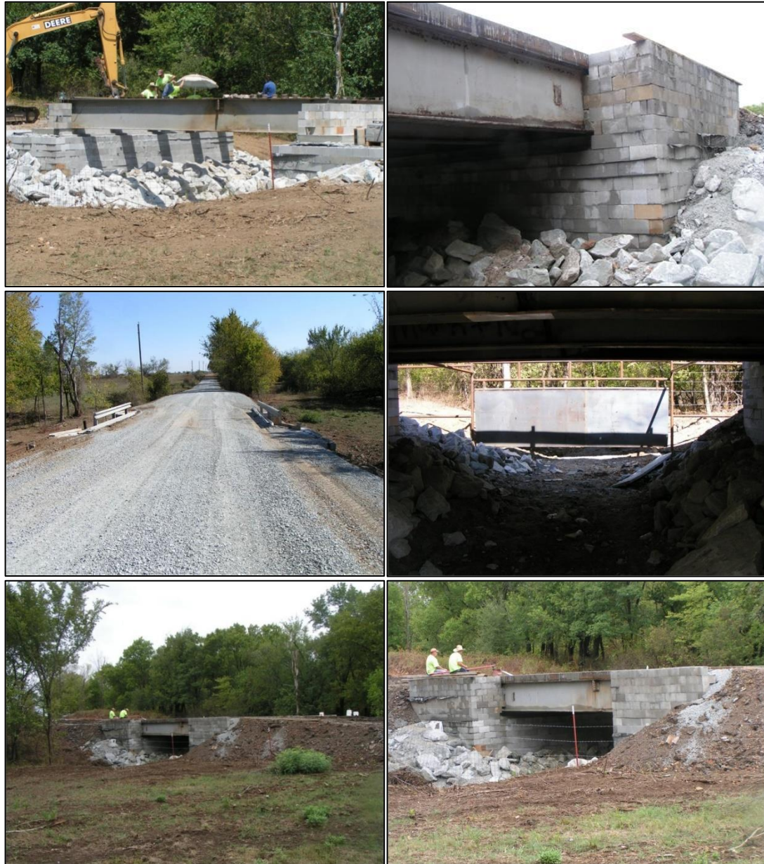
Figure 47: First GRS-IBS Bridge in Ottawa County, Oklahoma, built in 2013
