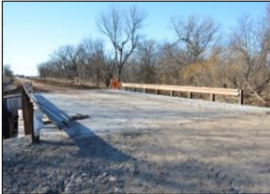
Figure 78: Completed Bridge No. 5 bridge (GRS-IBS) with sheet pile abutment facing
