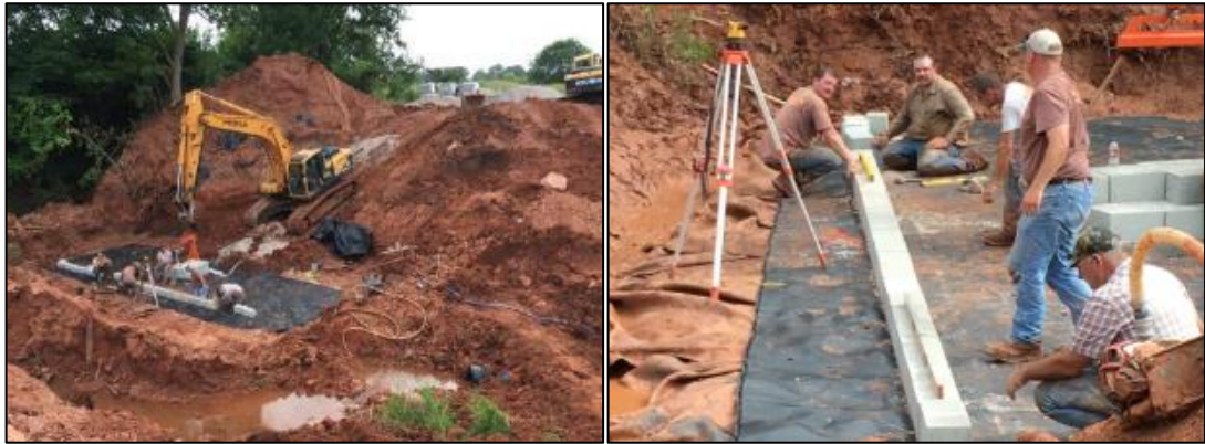
Figure 52: Placement of the first row of CMU blocks (Yates Bridge, 7/11/2016)
