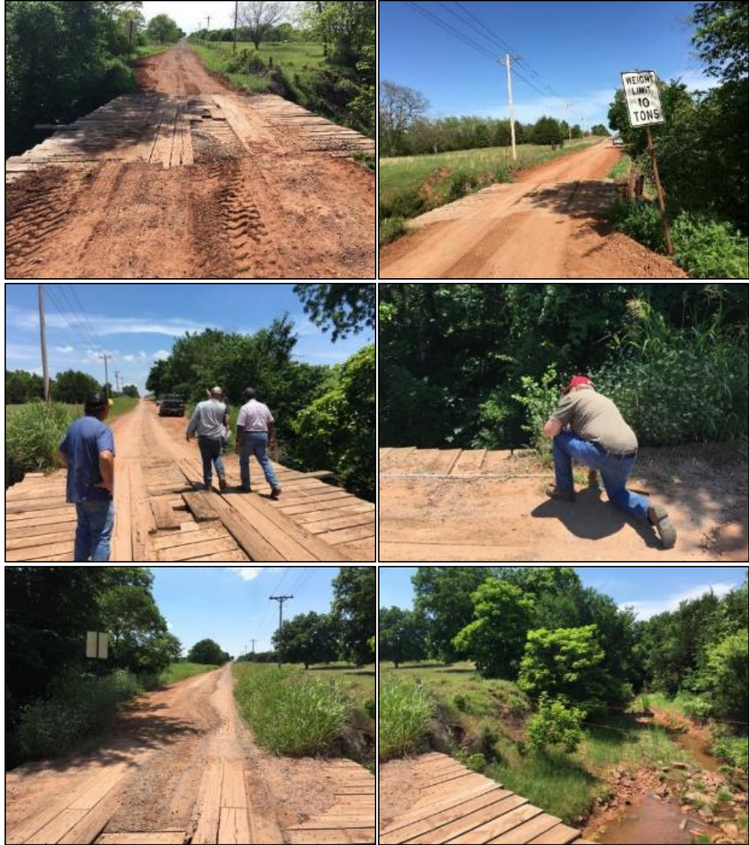
Figure 50: On-site preconstruction meeting on June 9, 2016 at Yates Bridge in Lincoln County
