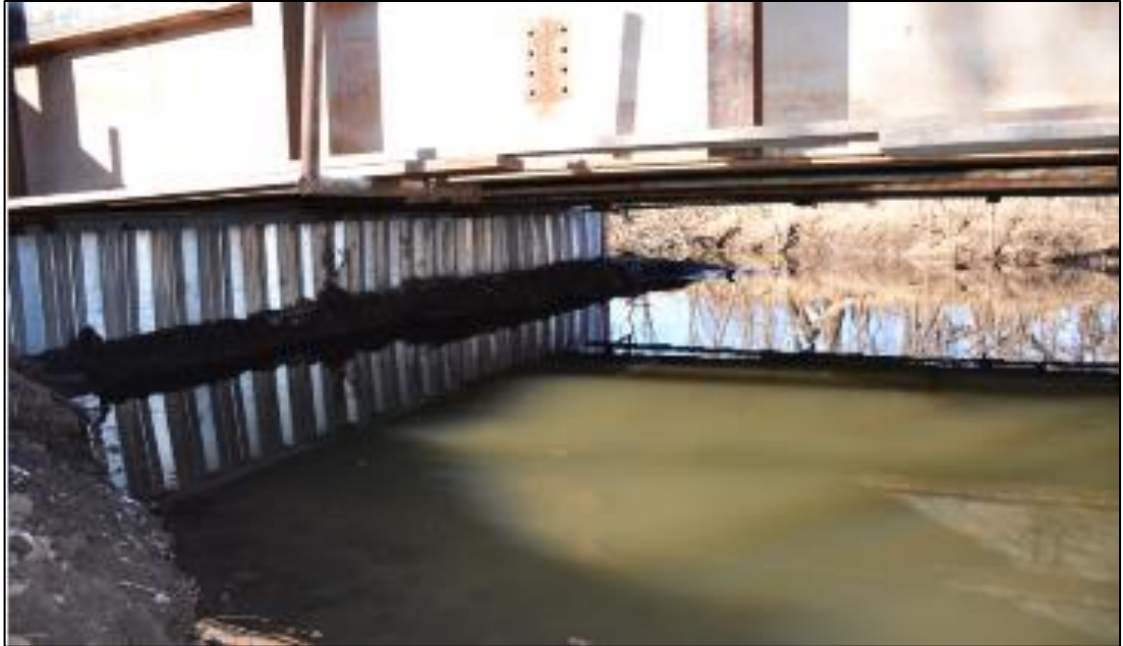
Figure 78: Completed Bridge No. 5 bridge (GRS-IBS) with sheet pile abutment facing
