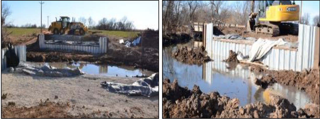
Figure 75: A GRS-IBS (Bridge No. 3) under construction near Blackwell in Kay County with sheet piling for the abutment facing
