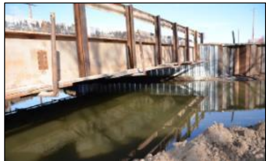
Figure 79: Completed Bridge No. 5 bridge (GRS-IBS) with sheet pile abutment facing
