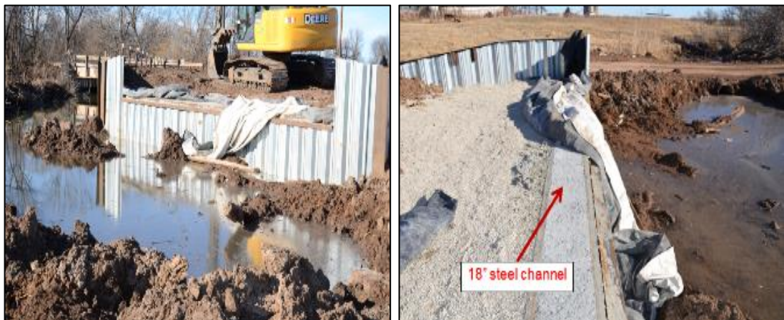
Figure 72: Bridge No. 3 - GRS-IBS under construction with sheet pile facing
