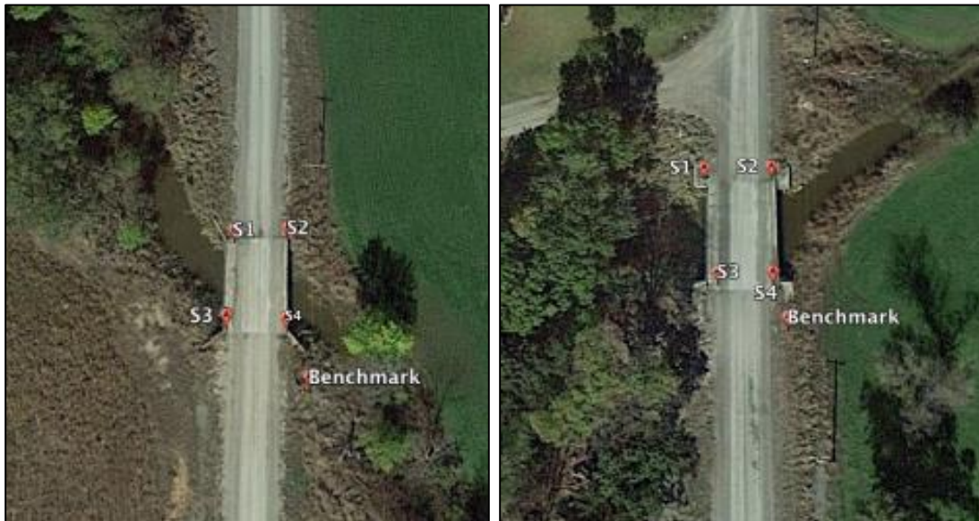
Figure 86: Bridges Nos. 1 & 2 with pilot survey points
