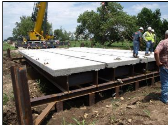
Figure 74: Bridge No. 6 - Bridge on conventional pile support under construction
