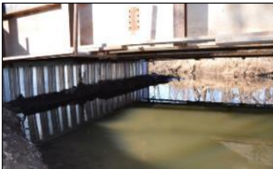
Figure 79: Completed Bridge No. 5 bridge (GRS-IBS) with sheet pile abutment facing
