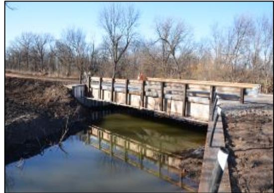
Figure 78: Completed Bridge No. 5 bridge (GRS-IBS) with sheet pile abutment facing
