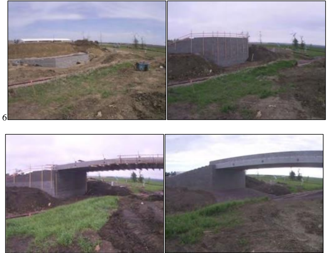
Figure 30: North abutment construction photographs for the CR-55 Bridge in Minnesota (Budge et al. 2014)
