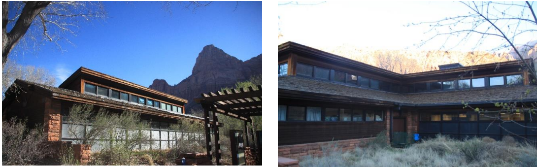
Figure 14: Clerestory windows in different height
